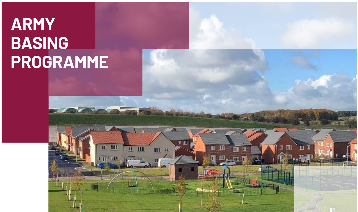
Army Basing Programme Larkhill Service Families Accommodation
