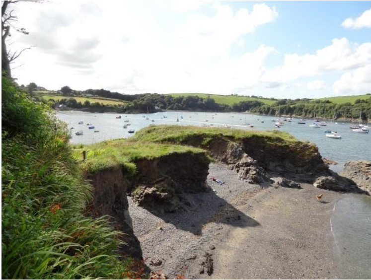
2012. More Magical views of the Herra from the coastal path, where it has now collapsed.
