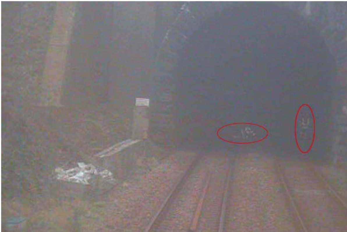
CCTV image from the approaching train (image courtesy of Transport for Wales)
