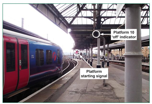
Figure 7: Platform 10 starting signal and 'off' indicator as seen from the rear of front vehicle
