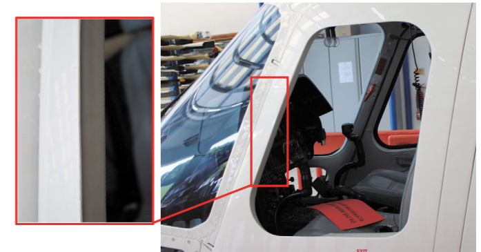
Window aperture of left cockpit door, showing no evidence of adhesive
