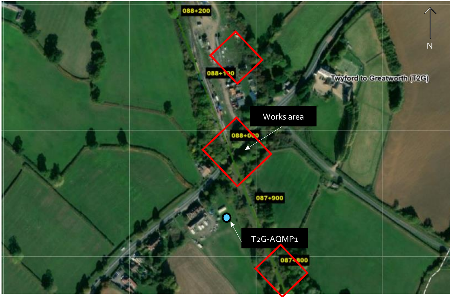
Figure 1: Worksite and monitoring locations during April 2021
