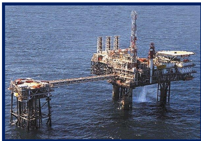
Figure 2. Ravenspur North Platform
