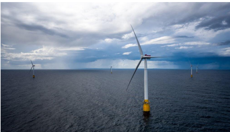
Figure 6: Hywind Pilot project installed turbines
