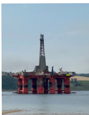
Transocean PBLJ commenced Phase II of MacCulloch decommissioning
