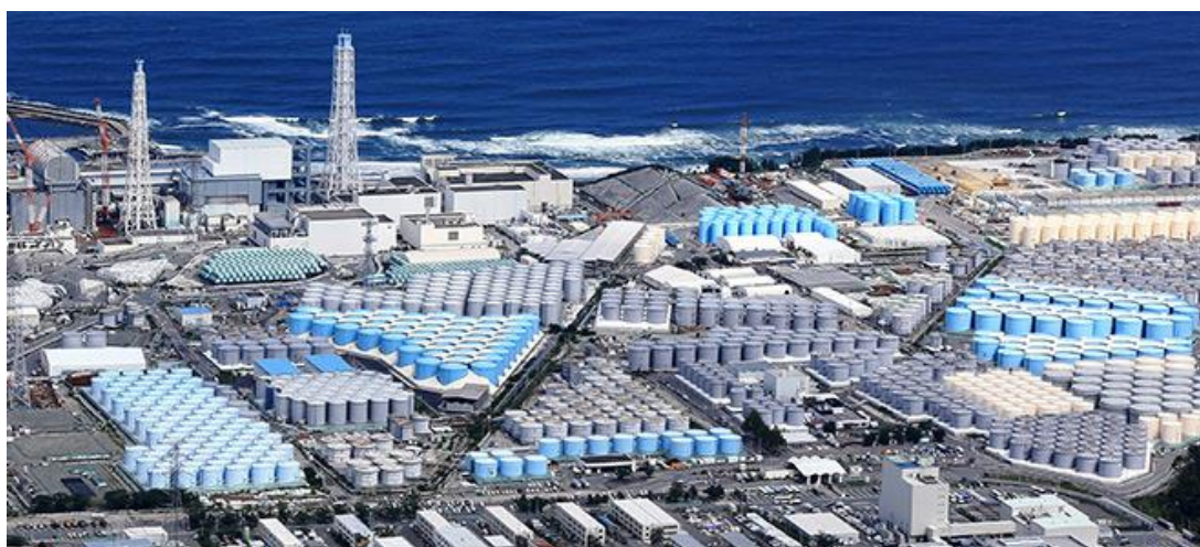
Figure A.3.2 Some of the tanks for the storage of tritiated water on the Fukushima Daiichi site.
