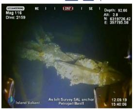
Figure 9.9-3: Mooring wire connection towards SAL anchor base
