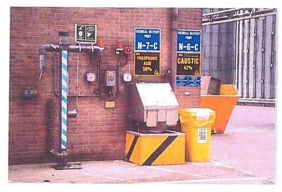
Plate 2: Chemical Fill Point without Bund and Unbunded Calcium Chloride Tanks
