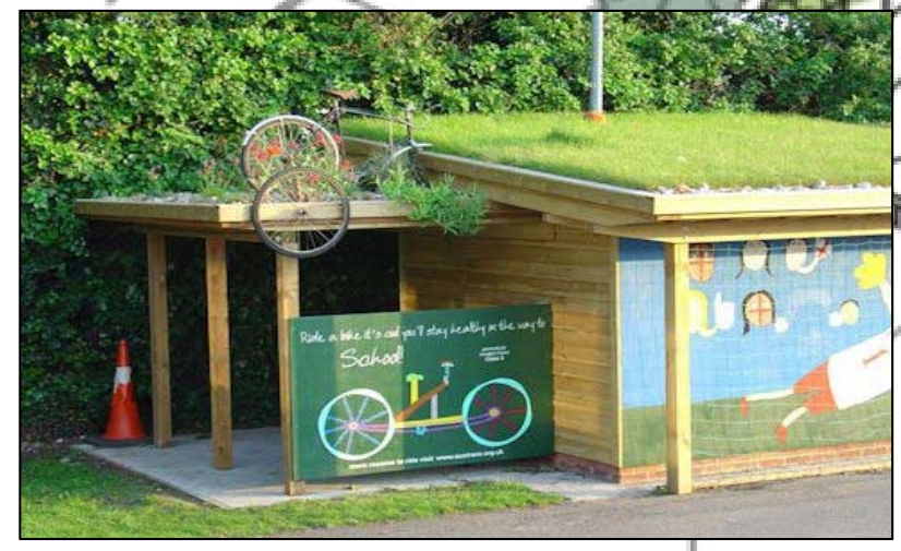
Green roof shades to cycle parking
