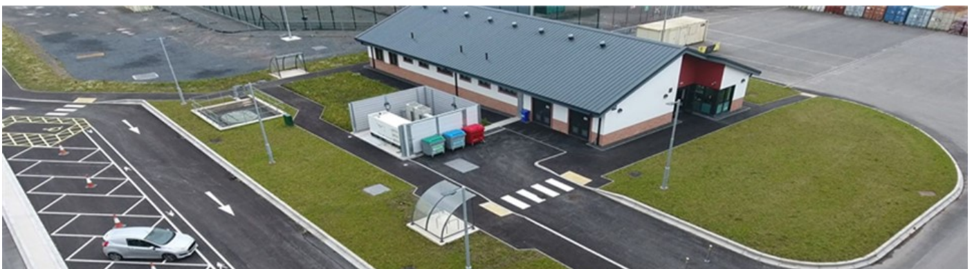
LLWR's new Site Emergency Control Centre (SECC) is now operational
