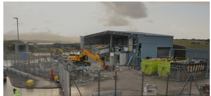
Magazine Retrieval Facility (MRF) being demolished
