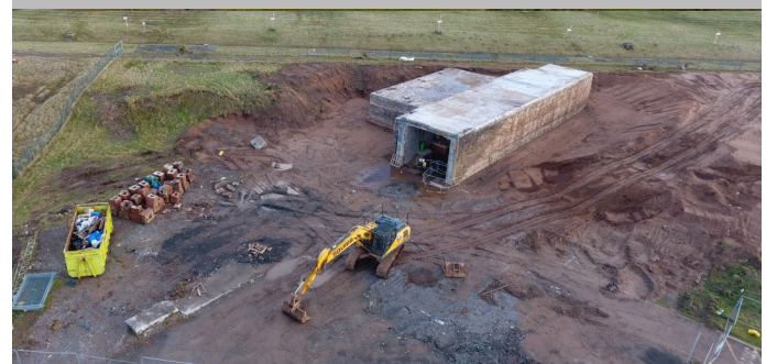
A magazine on the LLWR site is prepared for demolition
