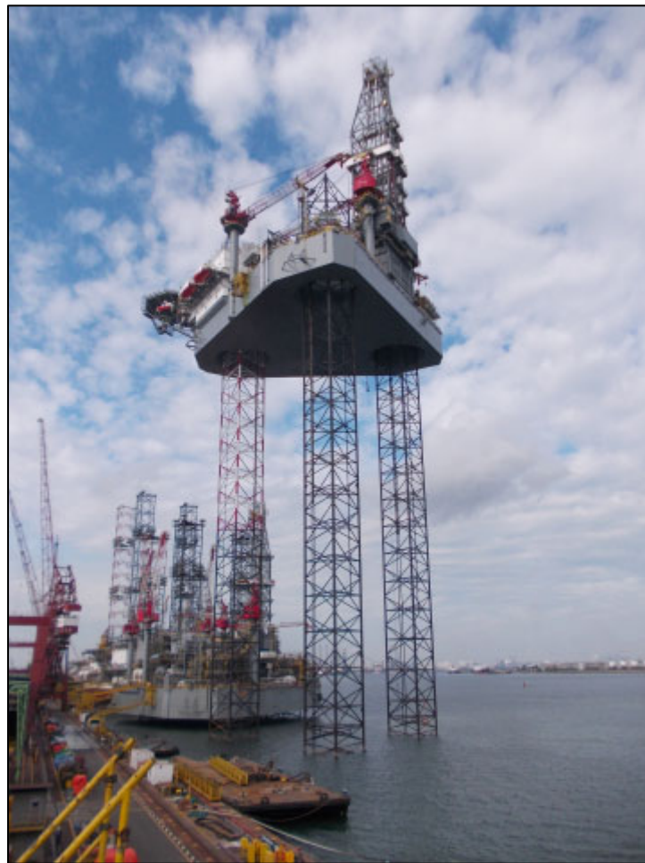
Figure 2-3 Example of jack-up MODU to be used for drilling at Tolmount East: ENSCO 120 series
