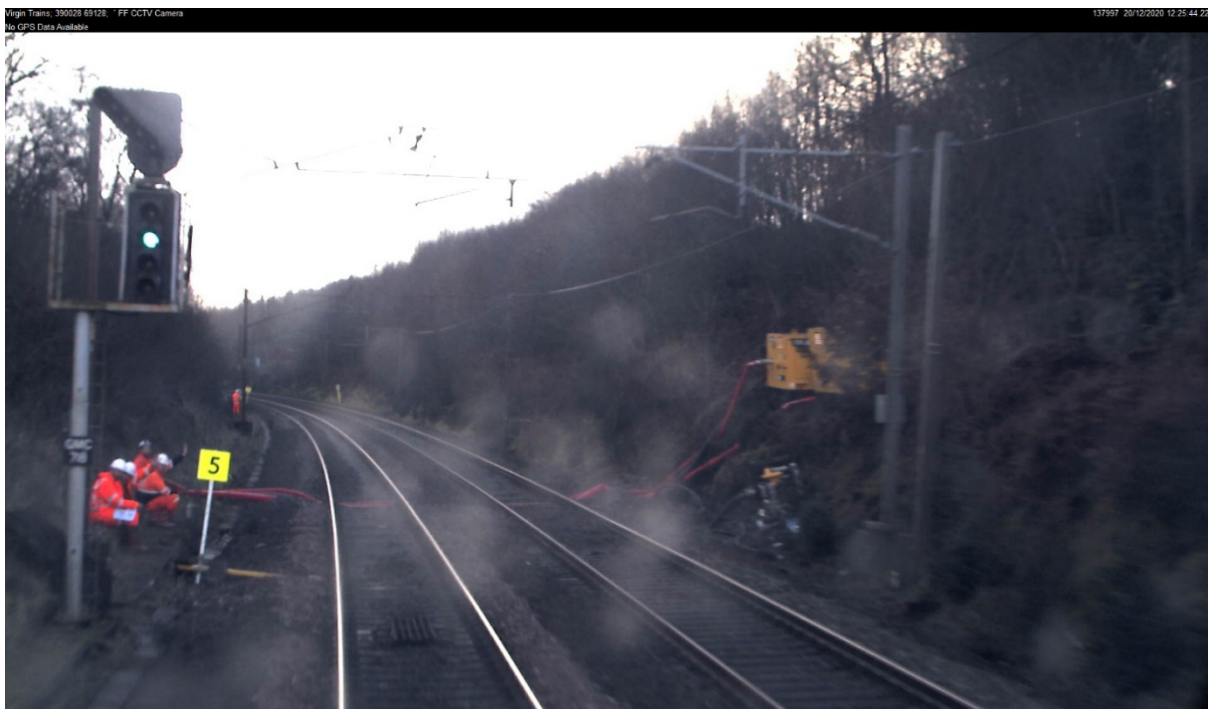
Forward-facing CCTV image from train 1M12 showing the speed indicator at the start of the ESR
