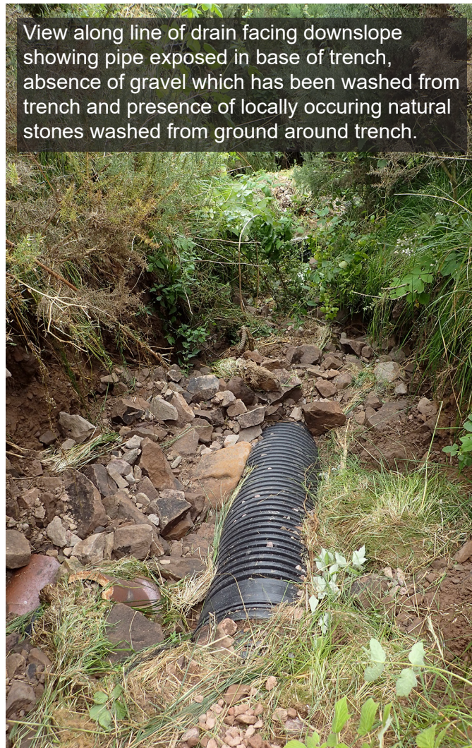
Figure 13: Drain with gravel washed out upslope of catchpit 18
