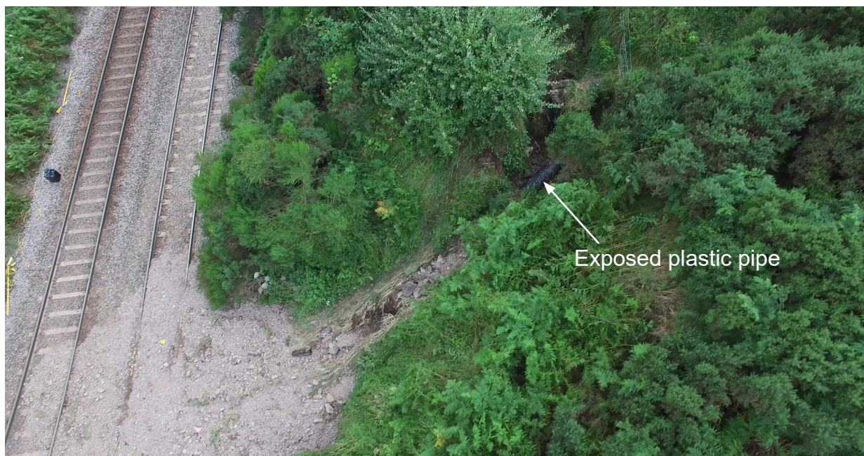
Figure 14: Drain downslope of catchpit 18
