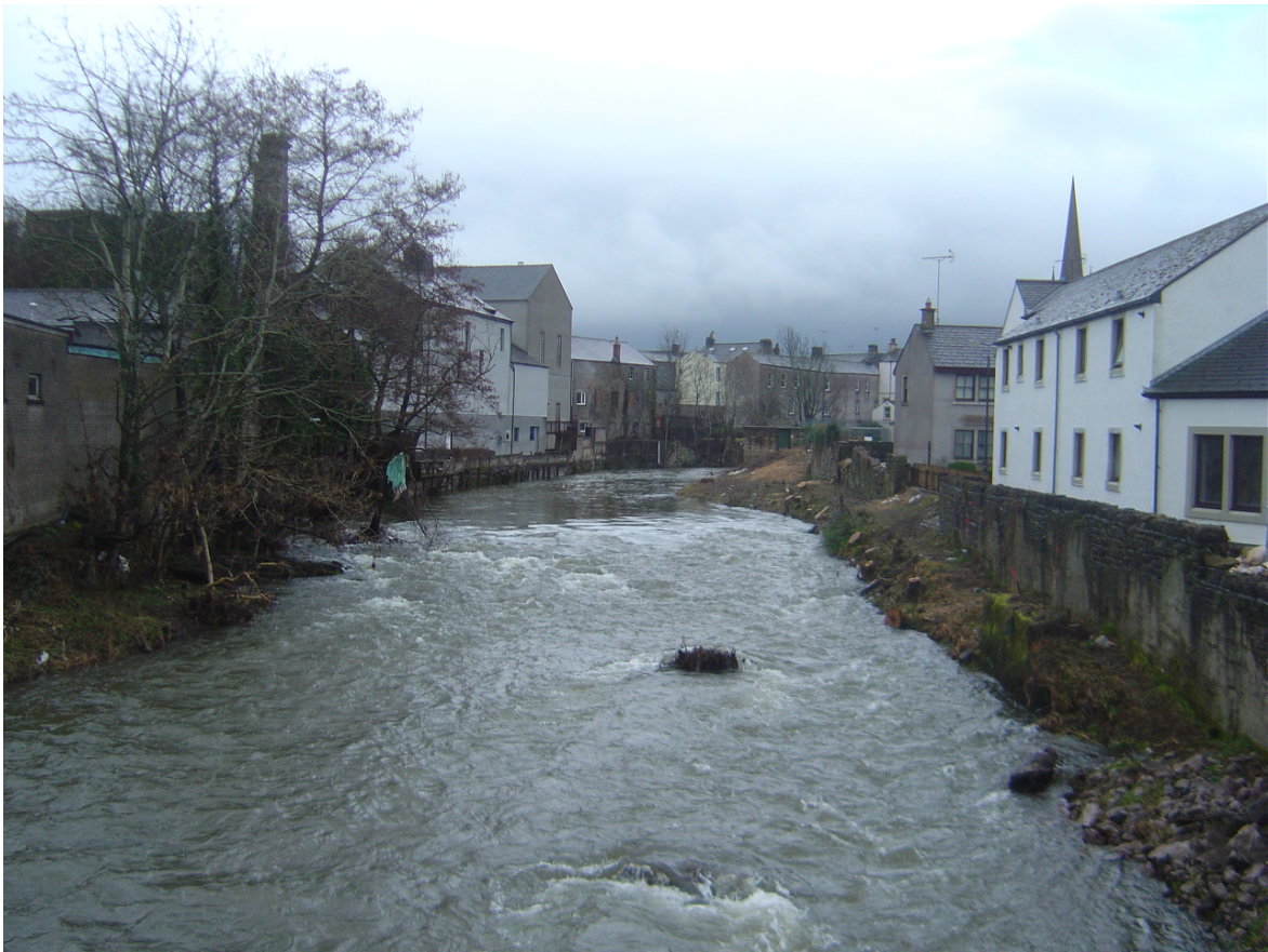
Figure 5 Example of urban confinement and, in the distance, constriction where development and flood protection walls along the River Cocker resulted in high stream power
