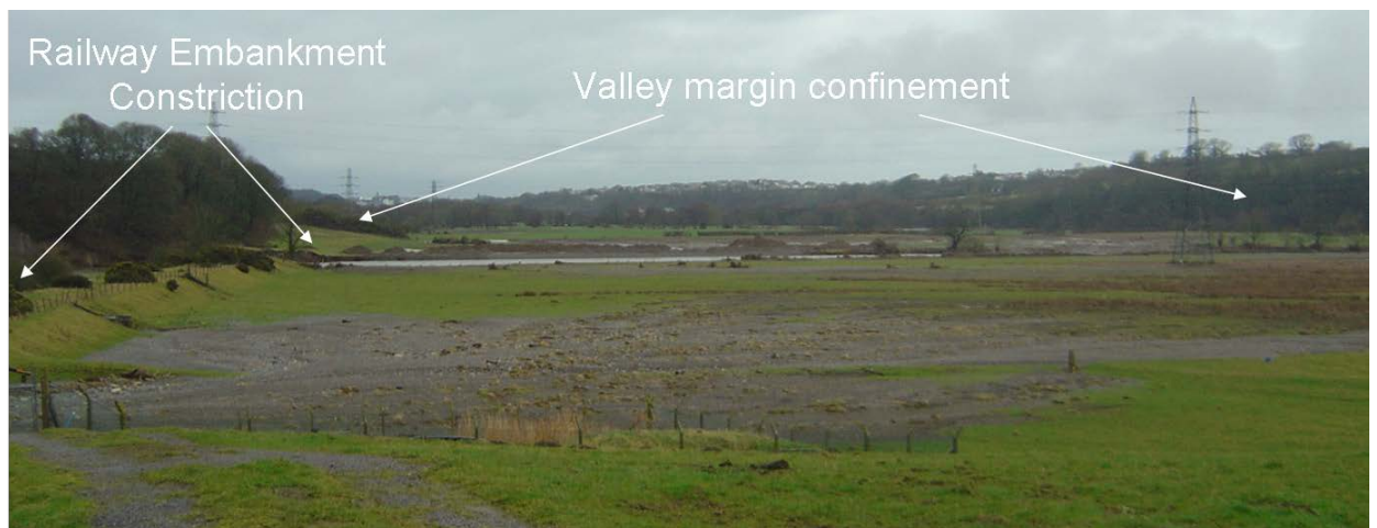
Figure 6 Example of a valley constriction created by a disused railway embankment crossing the flood plain and River Derwent downstream of Camerton
