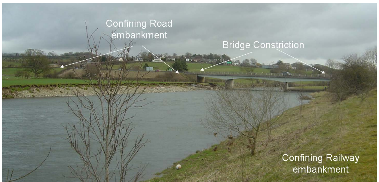
Figure 4 Examples of 3 sources of human activity that affect confinement and constriction during an extreme flood – Papcastle, Cumbrian Derwent
