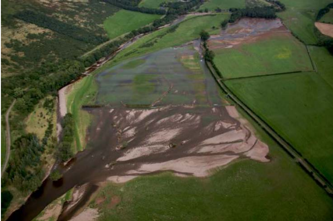
Figure 3-7 Embankment breach and changed course of the River Glen at Kirknewton (before reinstatement of channel in pre-event course to left, from Oughton and others (2009))
