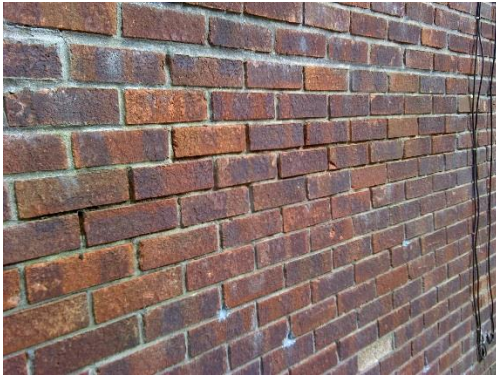
Eroded mortar
