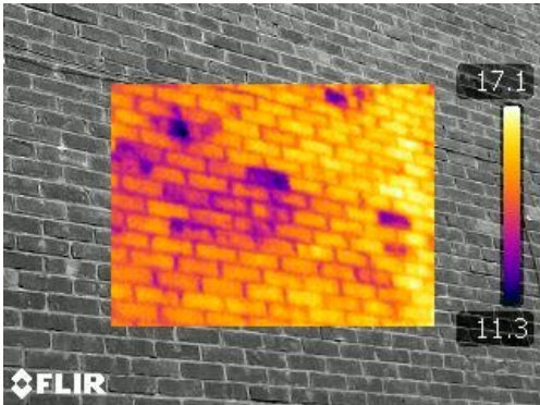
Elevated wetness in bricks caused by erosion or face damage
