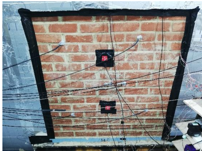
Figure 6: Position of the in-wall T&RH sensors seen from the internal leaf
