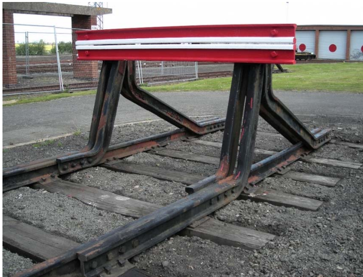
Figure 11.1 Buffer stop – traditional type
