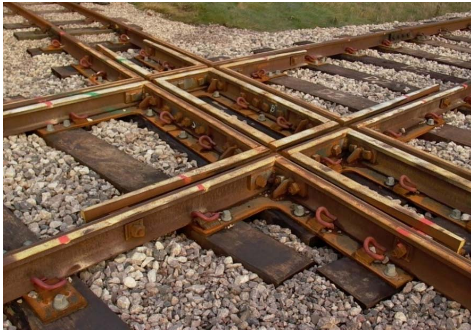
Figure 11.9 Standard/Narrow gauge grade crossing
