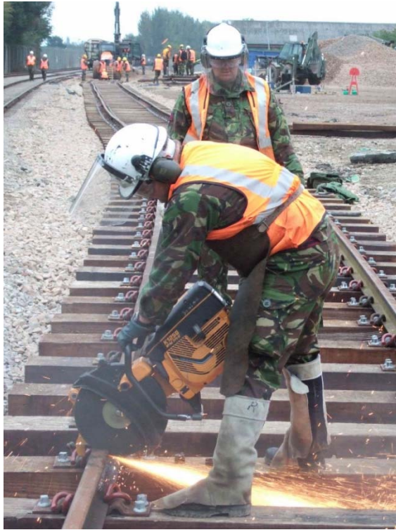
Figure 7.3 Cutting rails by disc cutter
