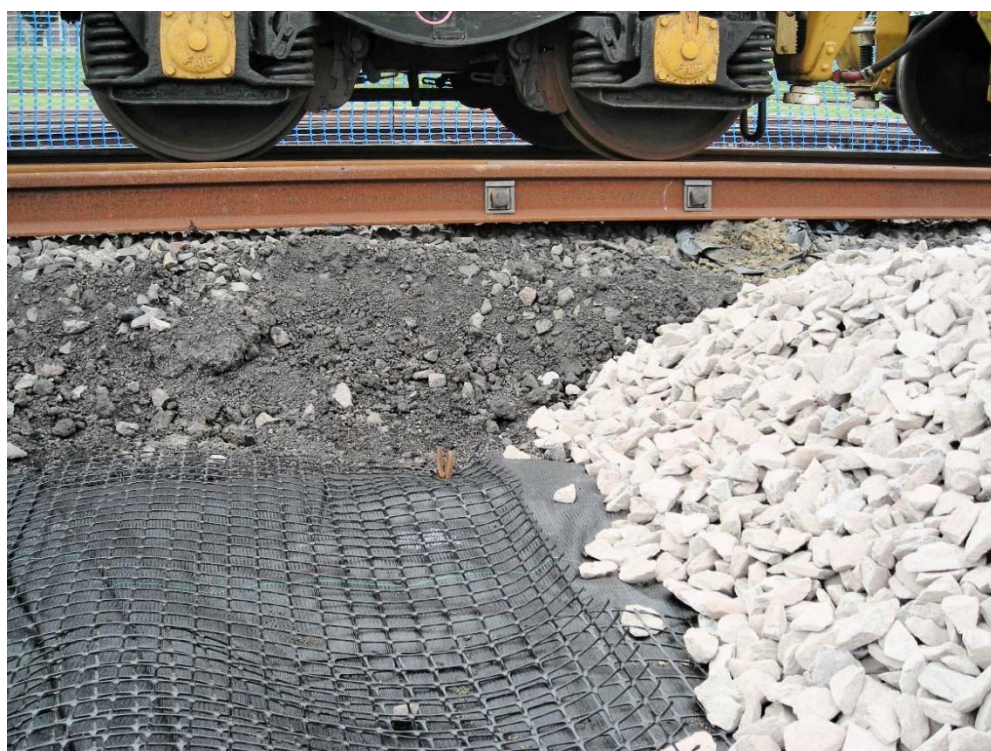
Figure 7.2 Geogrid over geotextile underlying new bottom ballast
