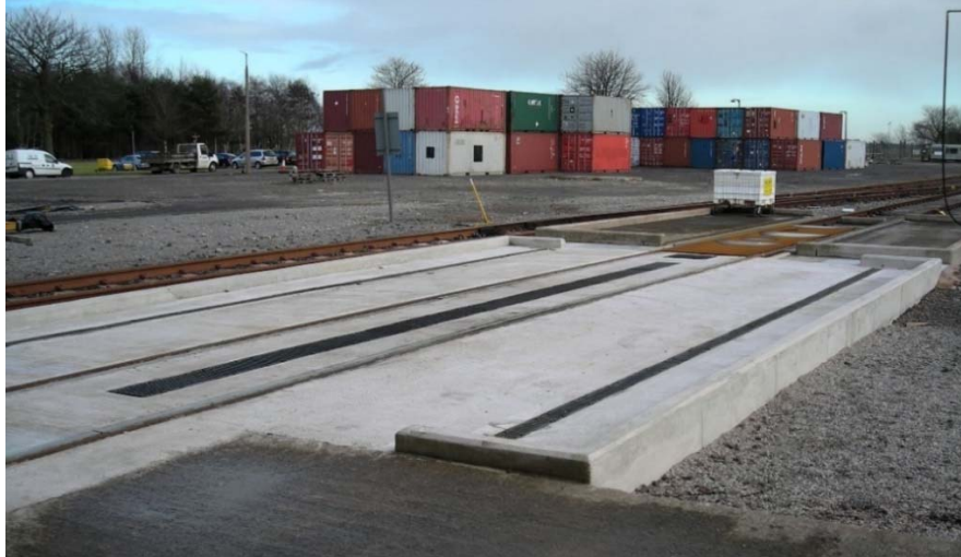
Figure 11.16 Wash down apron
