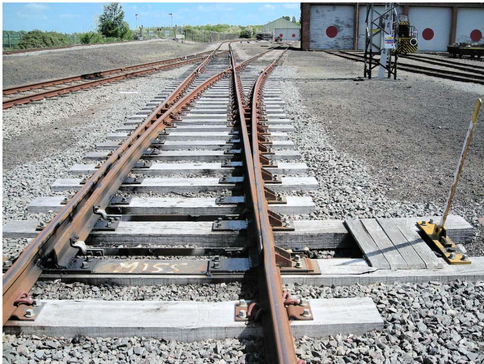
Figure 7.12 Switch element within a turnout
