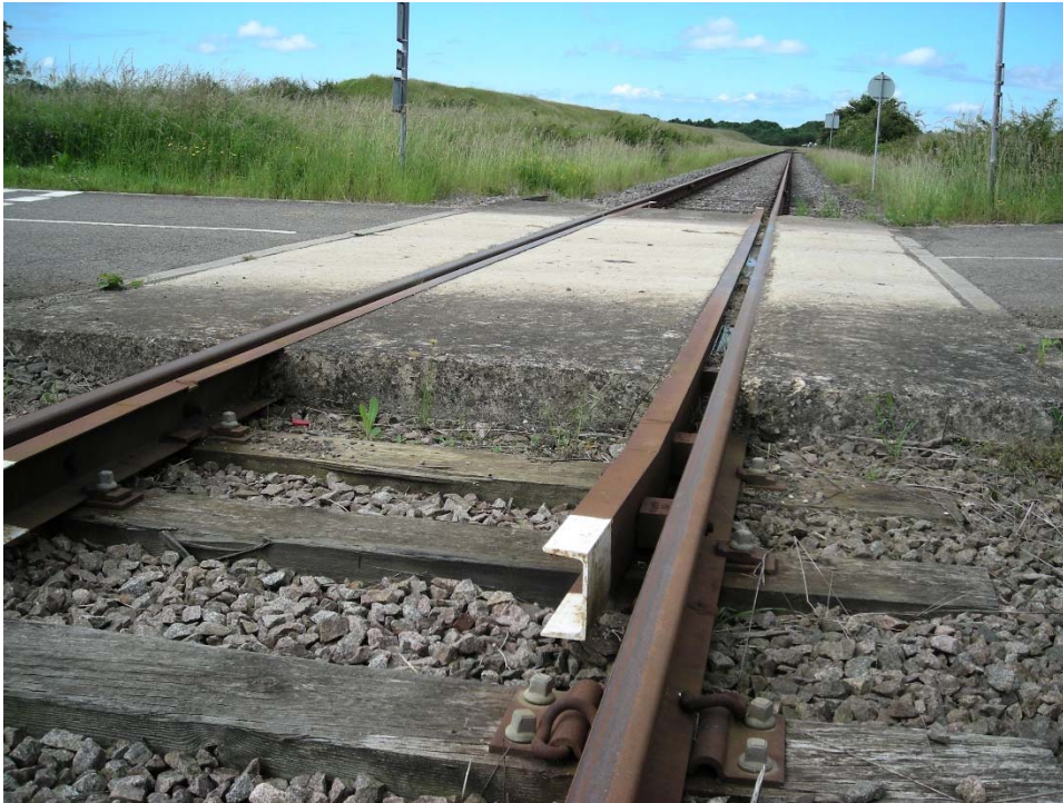
Figure 10.6 In-situ concrete paved type crossing
