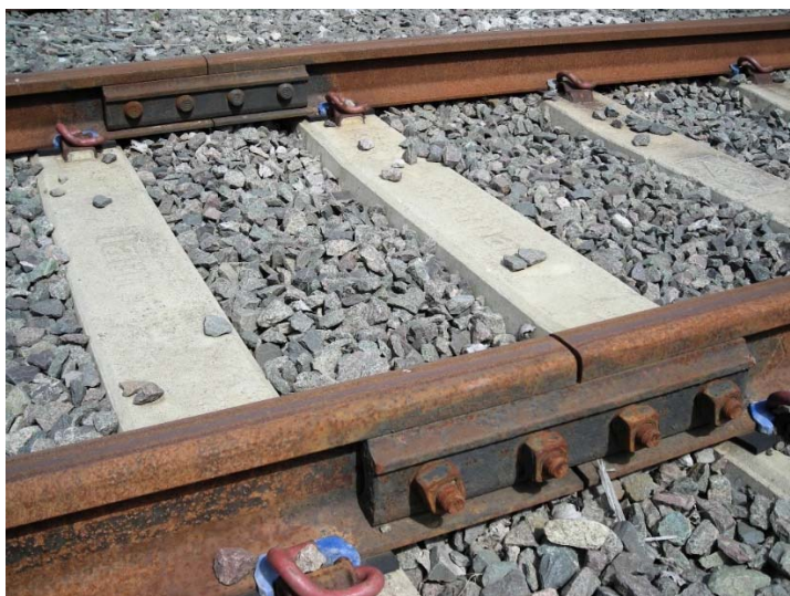
Figure 7.7 Fishplated joint
