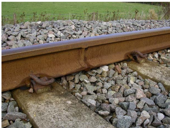
Figure 7.4 Alumino-thermic welded joint
