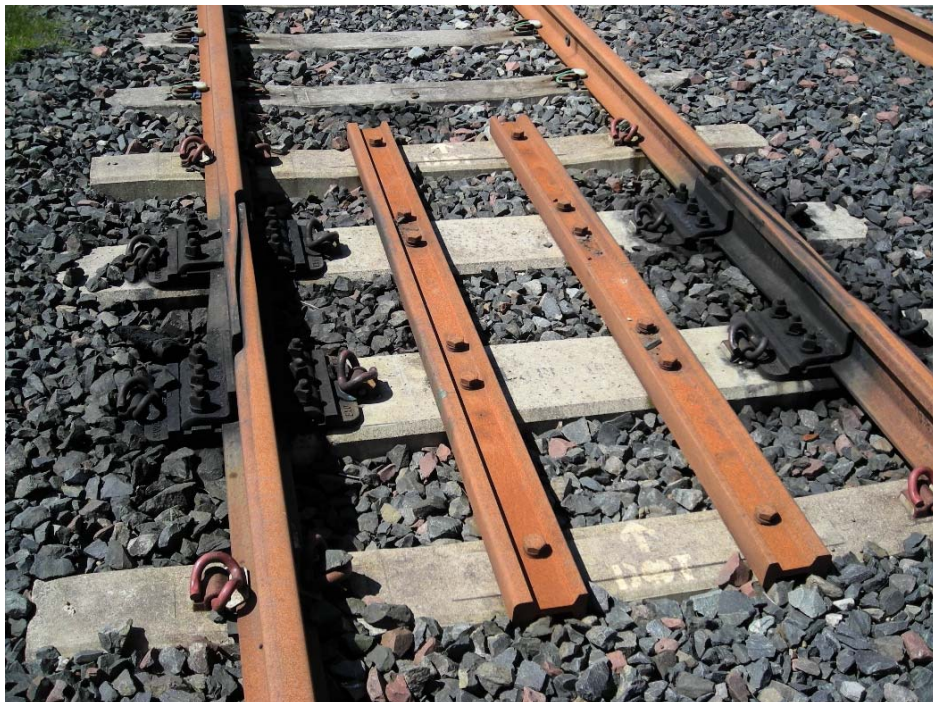
Figure 7.6 Typical adjustment switch in track
