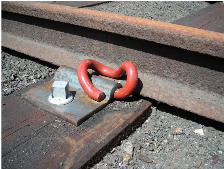
Figure 7.9 Pandrol clip PR401A with BS75R rail on wood sleepers
