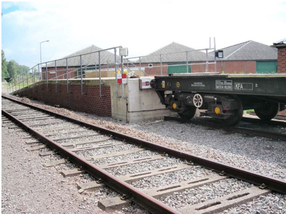
Figure 11.14 End loading ramp
