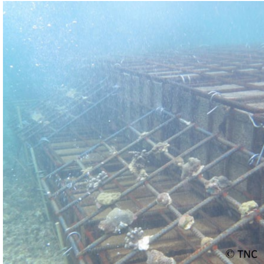
Figure 11. Complete breakwater structure provided by artificial reef in Grenville Bay, Grenada. Corals were transported from the original reef to increase biodiversity of the new artificial habitat (The Nature Conservancy).
