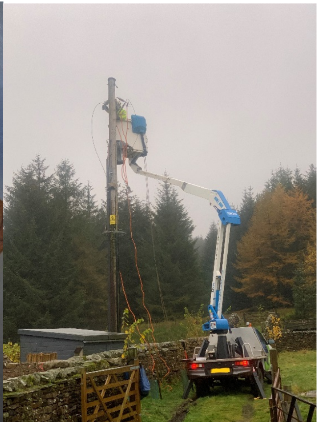
Figure 10: Engineers making the pole-mounted electricity transformer safe (image courtesy of F. Lumber).
