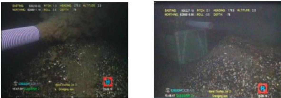
Figure 8-3: Photos of hose discharge and accumulation of cuttings at discharge point (DNV, 2017).
