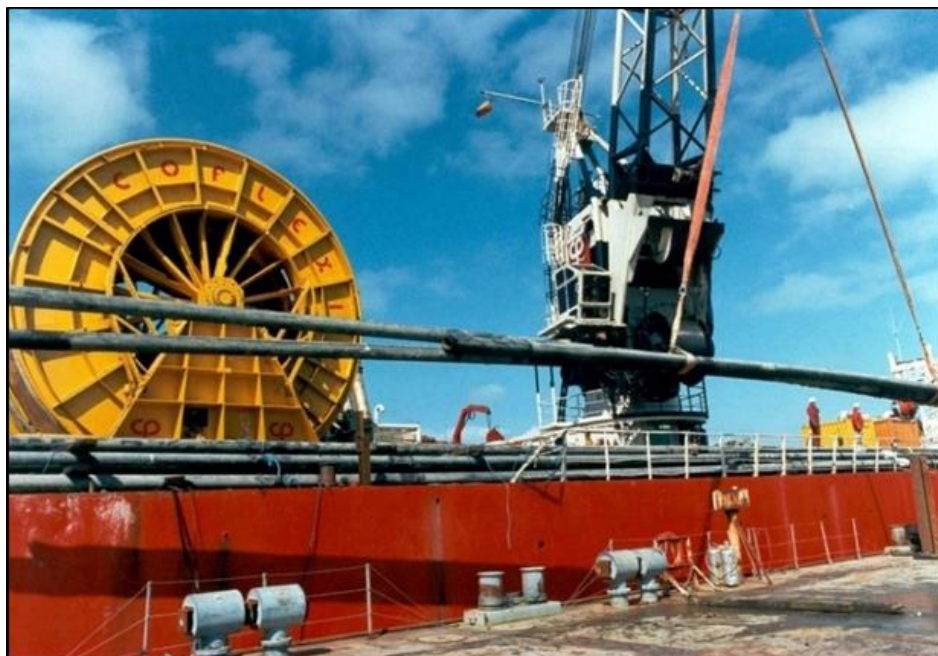
Figure 7: Pipeline Cut into Sections for Recovery
