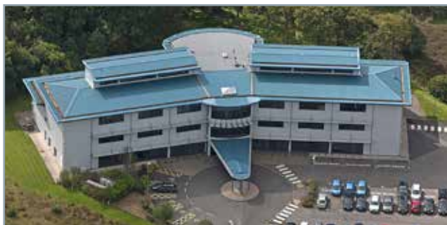
Reducing carbon across our offices as well as sites
