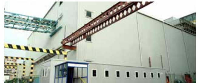
Magnox Reprocessing Plant - Sellafield
