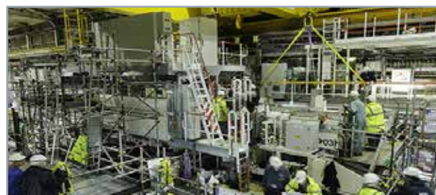
Emptying machine installation at the MSSS
