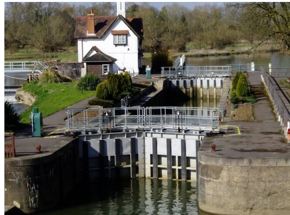
Figure 11.8 Modern steel lock gates
