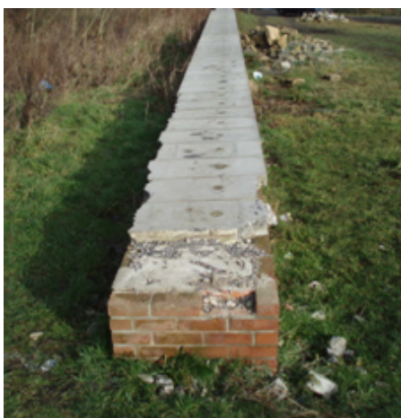
Figure 11.2 Example of resilience – a floodwall that survived a vandal attack
