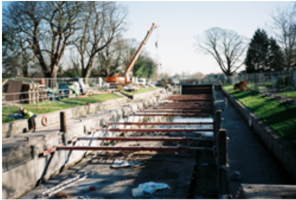
Figure 11.5 Penton Hook lock refurbishment
