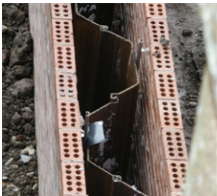
Figure 11.1 Example of vulnerability – a floodwall under construction, awaiting capping slabs
