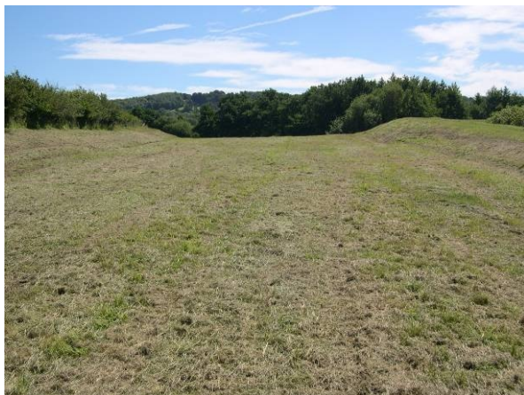
Figure 10.13 Plain grass spillway
