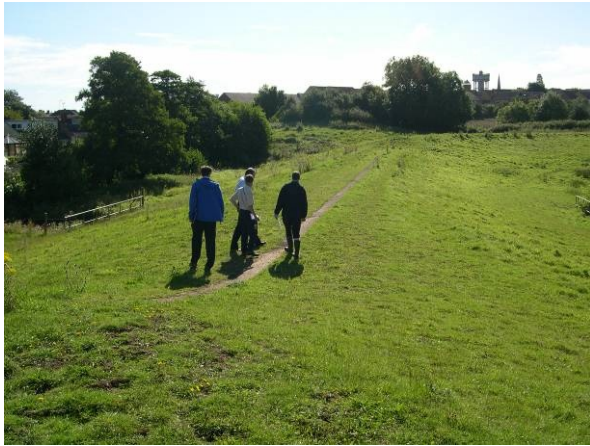
Figure 10.14 Reinforced grass spillway
