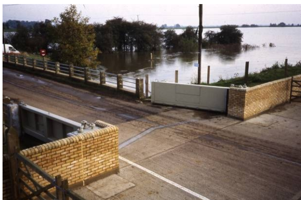
Figure 9.8 Gates to provide road access
