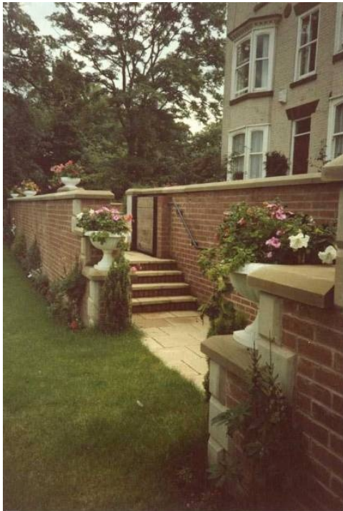
Figure 9.17 Floodgate in a brick-clad sheetpile floodwall, Boroughbridge (Yorkshire)
