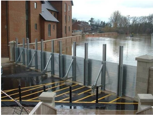
Figure 9.15 Frankwell flood alleviation scheme, Shrewsbury (River Severn)
