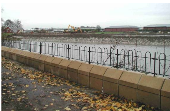
Figure 9.19 Precast block floodwall
