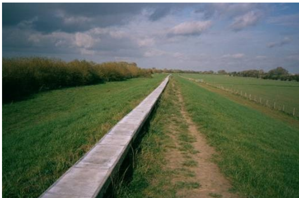
Figure 9.10 Floodbank with crest wall
