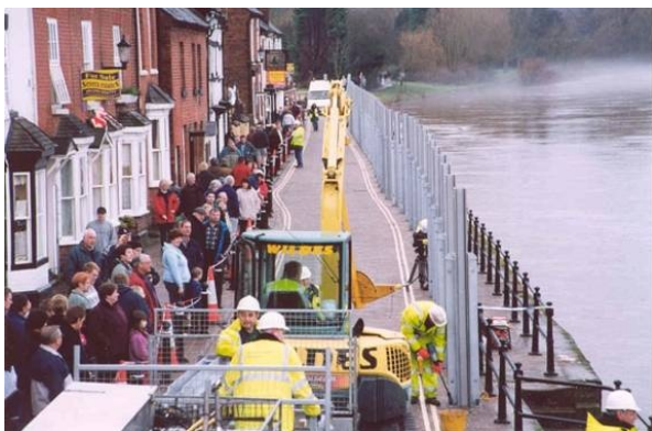
Figure 9.16 A demountable defence being erected at Bewdley (River Severn)
