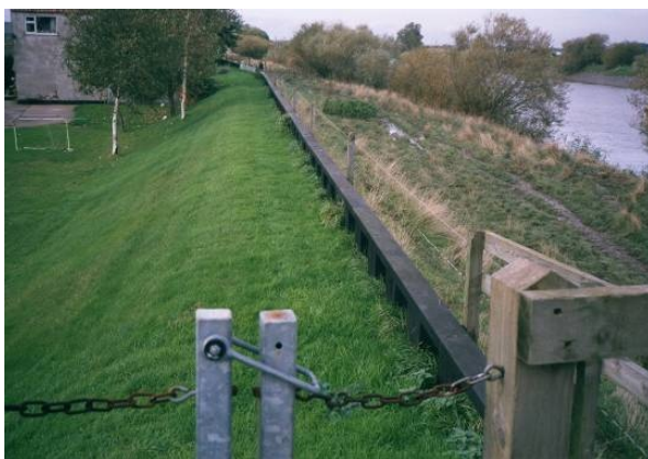
Figure 9.11 Flood embankment with sheetpile wall
