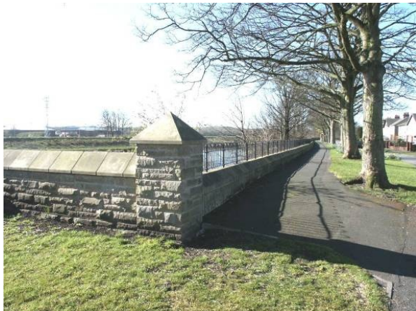
Figure 9.18 Is it a floodwall?
