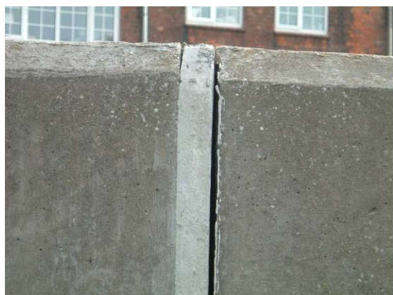
Figure 9.7 Joint in concrete floodwall
