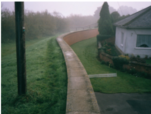
Figure 9.5 Flood embankment combined with floodwall
