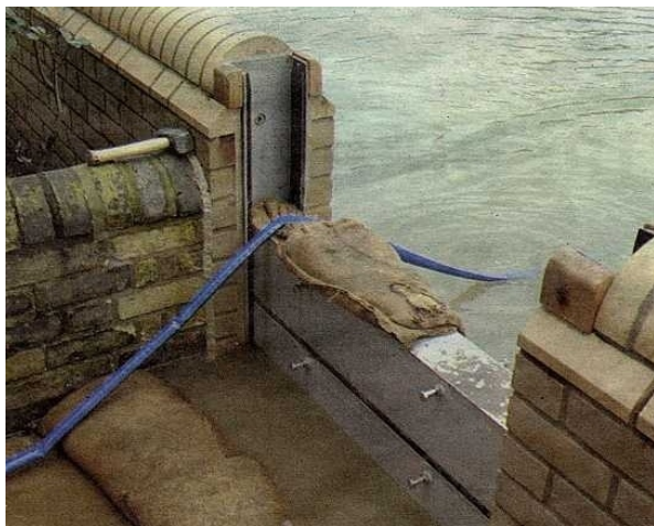
Figure 9.9 Removable defence in a floodwall in Cambridge
