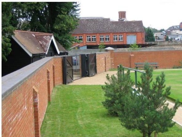
Figure 9.6 High floodwall with large floodgate for access – Frankwell, Shrewsbury
