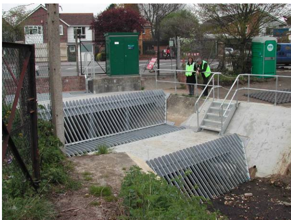
Figure 8.26 Well-designed screen
