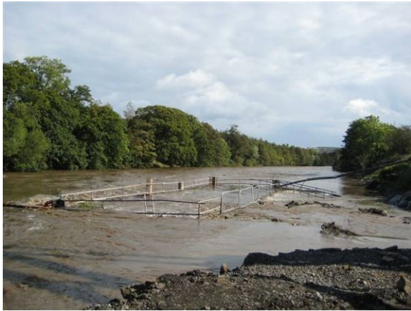
Figure 8.27 Cofferdam in flood conditions
