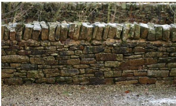
Figure 5.6 Localised floodwall in a sensitive, rural village setting
