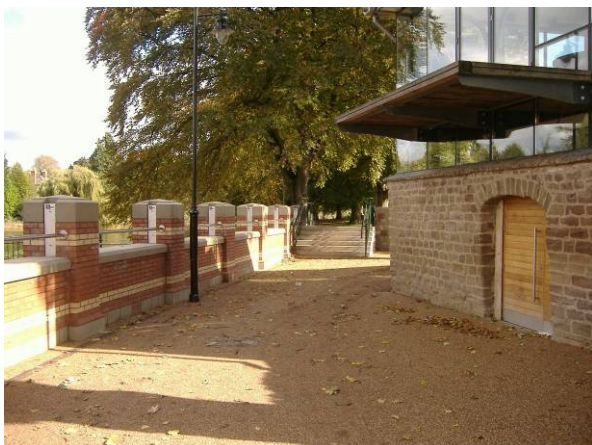
Figure 5.7 Localised floodwall in a sensitive, urban setting
