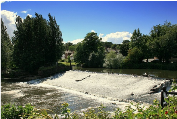
Figure 5.10 Weirs and sluices
