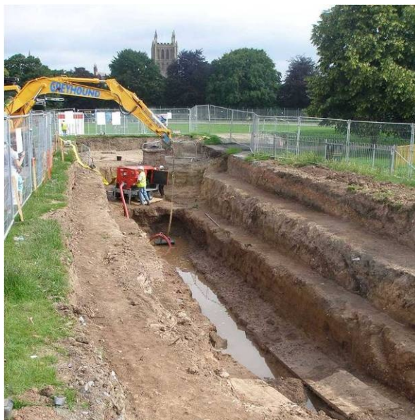
Figure 5.17 Major construction activity
