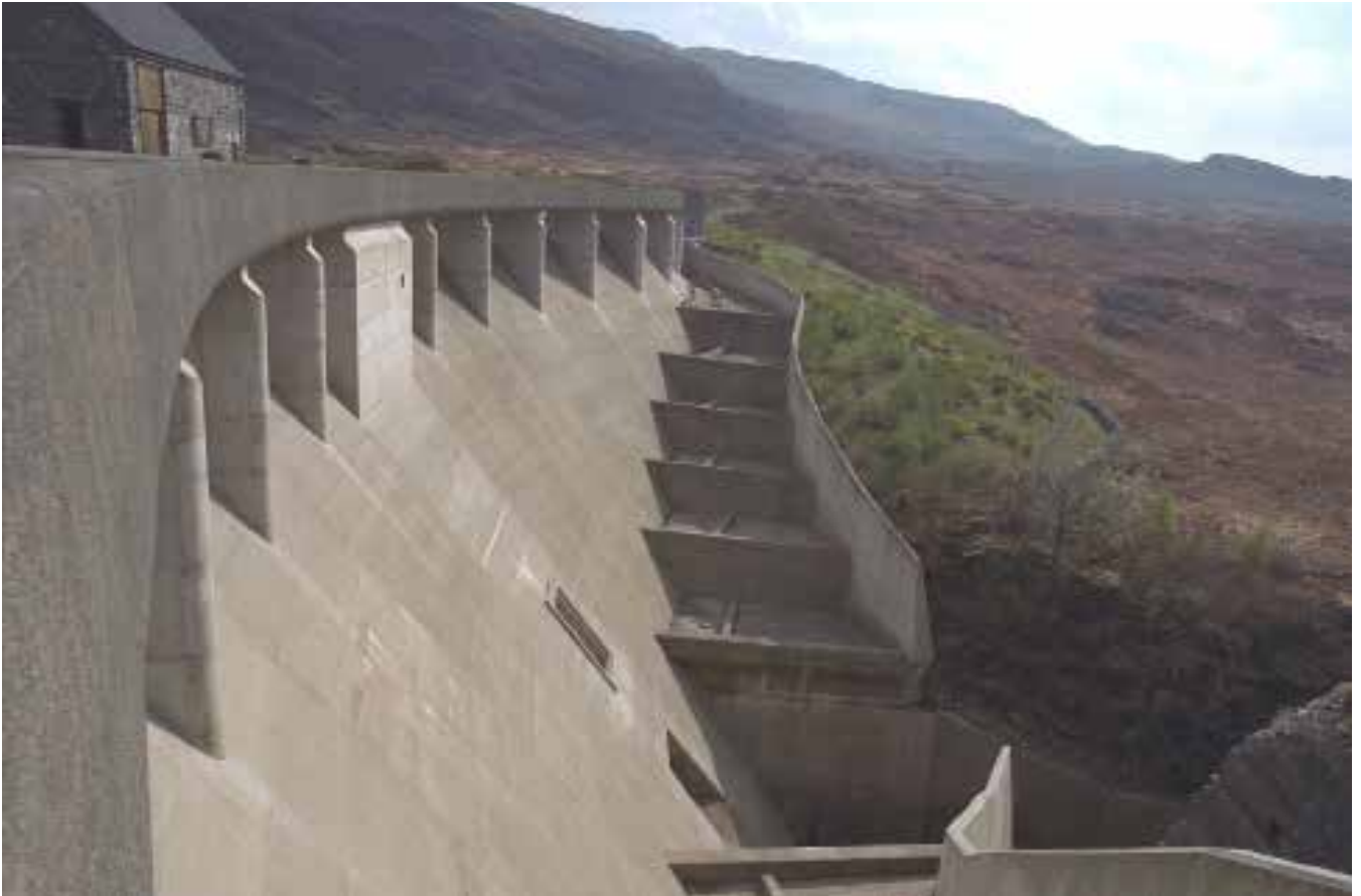
Maentwrog hydro-electric power station
