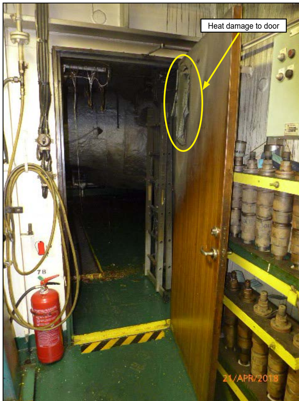
Figure 3: Purifier room door
