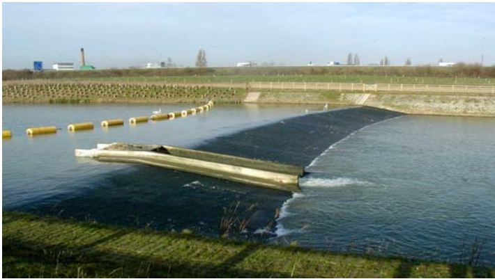
Figure 2.32 Weir on the Jubilee River
