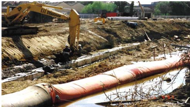
Figure 2.17 Temporary diversion of a stream
