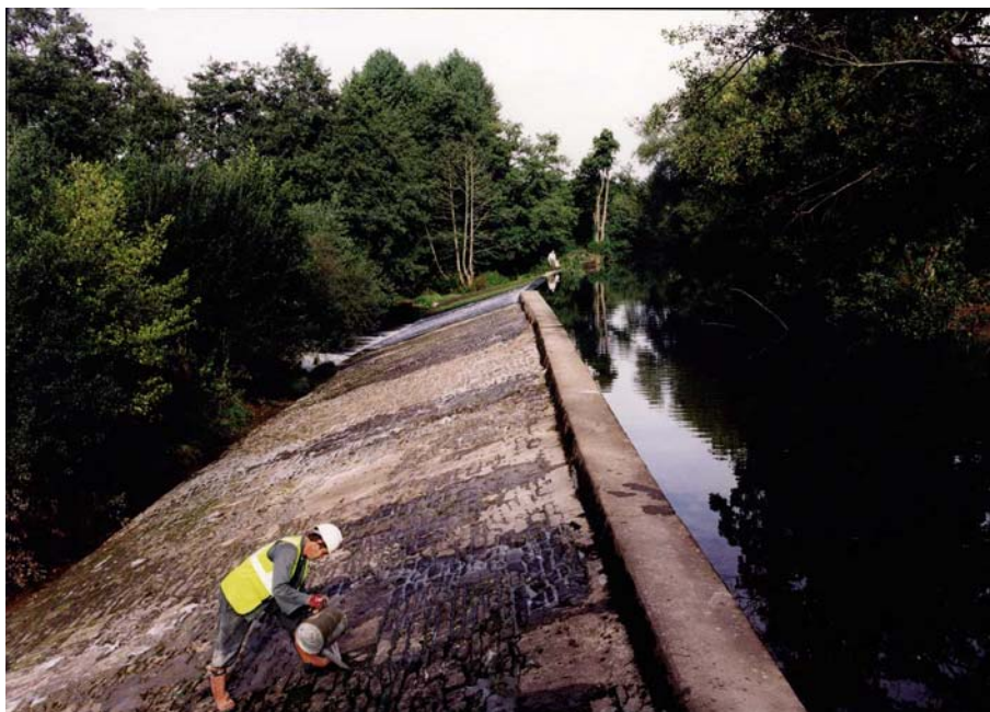
Figure 2.14 Repairs to mortar joints in a masonry weir
