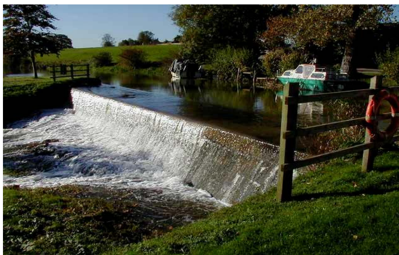
Figure 2.6 Dangerous side weir?
