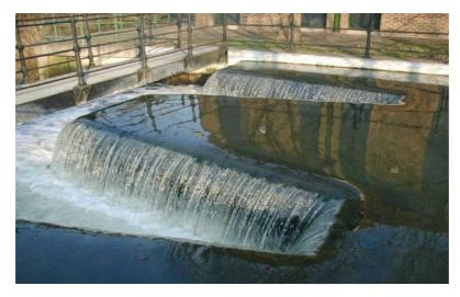
The labyrinth weir has a long crest length in a relatively short overall width. It is therefore good for reducing upstream water level variation in low to moderate flows. In flood flow conditions, the labyrinth effect is diminished, and the weir will tend to perform as a broad-crested weir with a crest length equal to the width of the channel.
