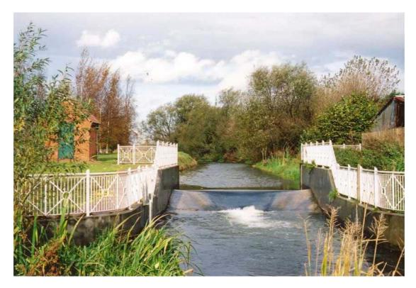
A modern discharge monitoring weir of the flat-vee type. This type of weir is often favoured for its accuracy of flow measurement and suitability for both low and high flows. It is one of the best weirs for sediment conveyance, but tends to make fish migration difficult. Note that it is possible to create an attractive gauging weir that sits well in its surroundings.
