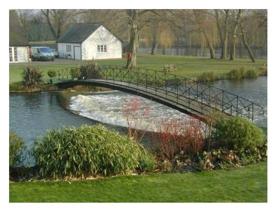
Not all weirs can be designed to enhance the visual environment as much as this graceful structure with its arching form and matching elegant footbridge, but even a little extra thought at the planning and design stages can yield significant environmental benefits. Note that this weir has two fish passes, one on either flank.
