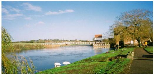
A former mill weir at Tewkesbury now replaced by a tilting gate allowing precise control of upstream water level. Note that works of this nature can readily blend in with an attractive landscape. The weir is on the right of the picture, and is indistinguishable from a conventional weir.
