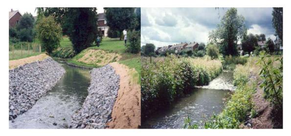
The creation of a riffle in a small urban brook can look quite stark immediately after construction, despite the use of natural materials (rock). However, as the second photograph (taken one year later) shows, such works soon blend into the environment.
