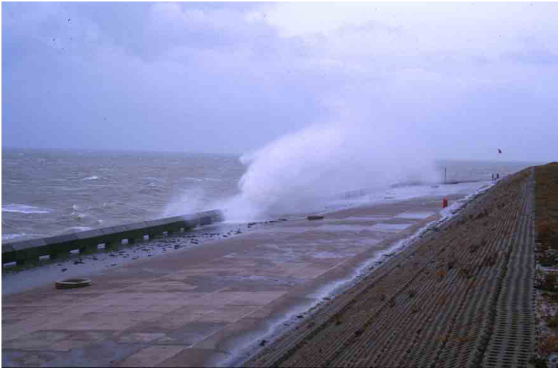
Figure 6 Example of overtopping rate of about 0.3 l/m/s at Samphire Hoe (photo HR Wallingford)
