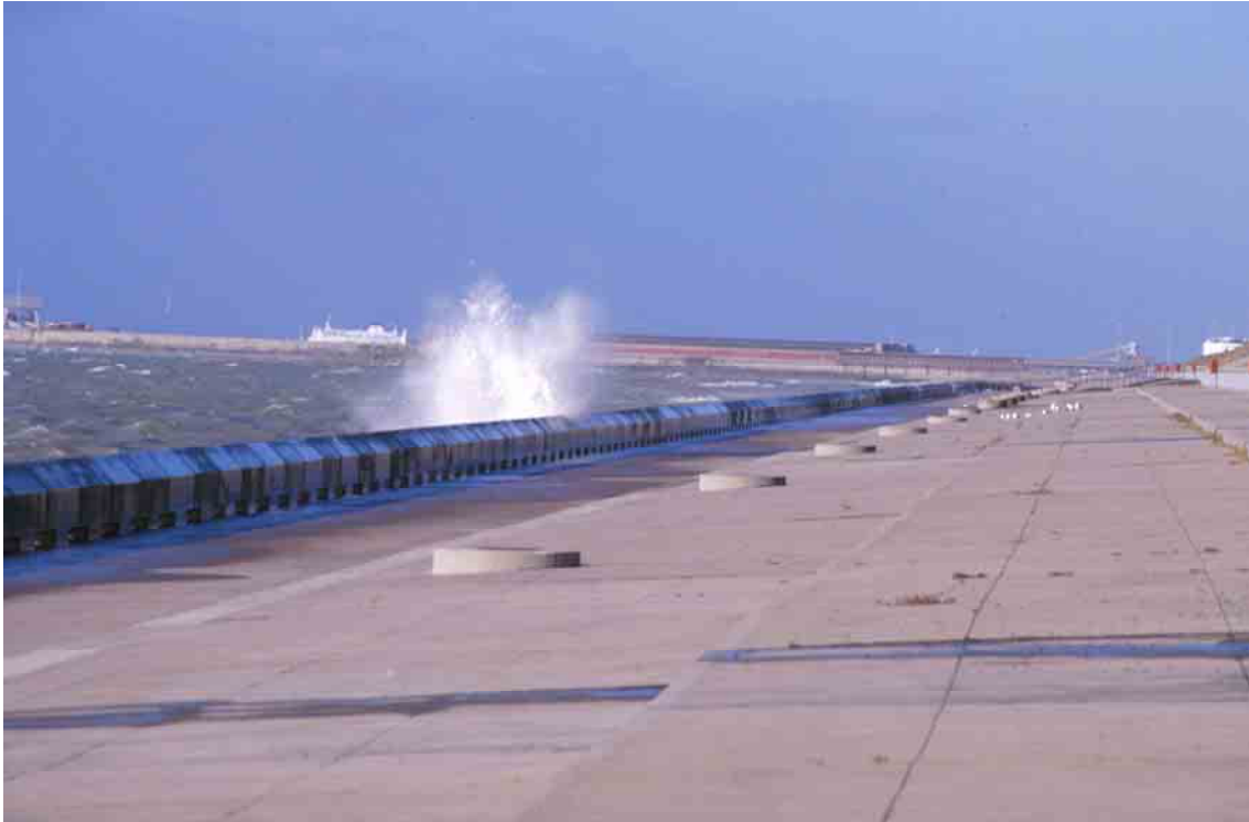
Figure 5 Example of mean overtopping rate of about 0.03 l/m/s at Samphire Hoe (photo HR Wallingford)
