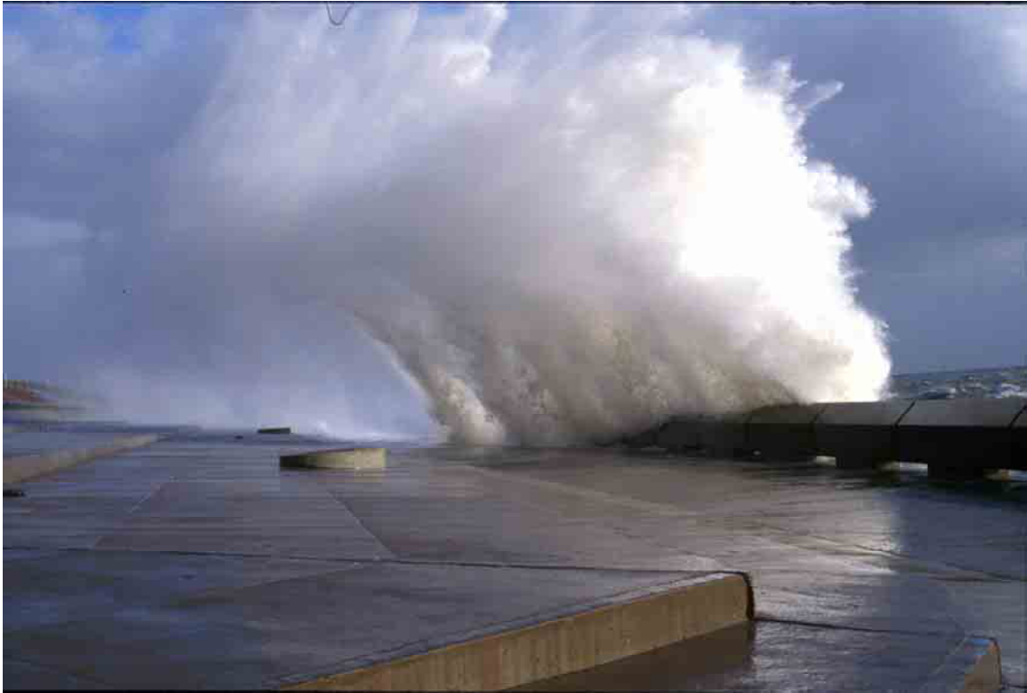
Figure 7 Example of peak overtopping occurring during mean overtopping rate of about 3.0 l/m/s at Samphire Hoe (photo HR Wallingford)
