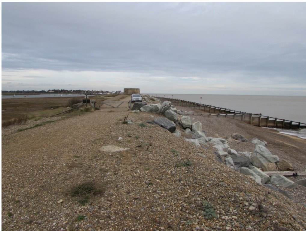
Figure 0.18. The artificially profiled shingle ridge south of the Martello Tower, showing groynes and rock armour protection (Photo Courtesy of K. Pye).
