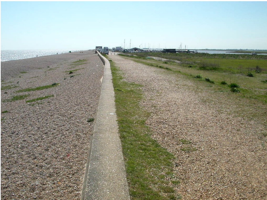
Figure 5.1: The concept of coastal squeeze, although most commonly applied to saltmarshes, can also apply to other coastal habitats such as shingle beaches that are backed by structures such as sea walls.
