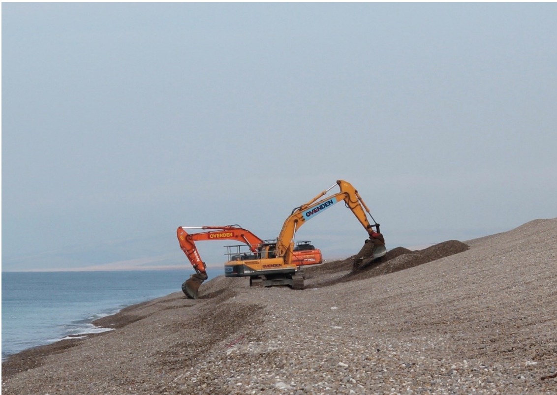
Figure 6.4: Beach reprofiling at Chesil Beach, Dorset following 2014 winter storms. Sediment is moved from the lower to the upper beach, to maintain the crest elevation which prevents breaching and natural landward transgression.
