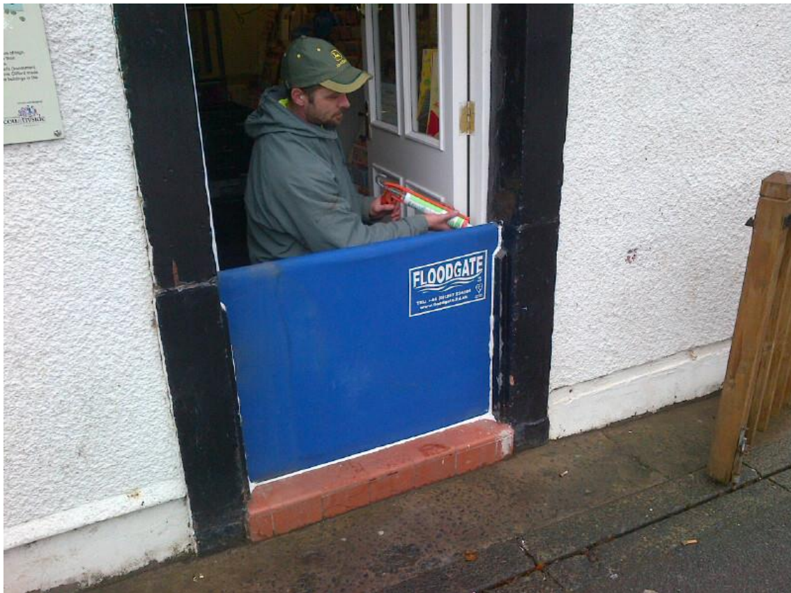
An example of a flood gate (Source: Environment Agency)
