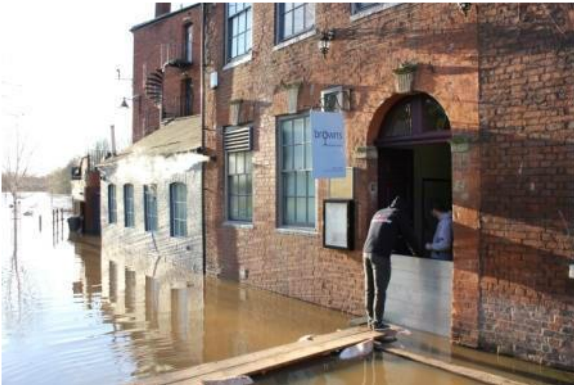
Property flood resilience measures in operation Worcester during 2012 Floods (Source: Environment Agency)
