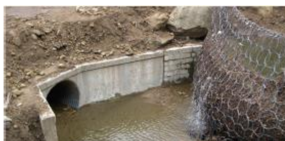
Figure 4.4 Flexible net barrier upstream of a culvert
