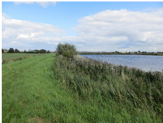
Figure 39: Example of “Satisfactory” Condition (Anglian Region)
