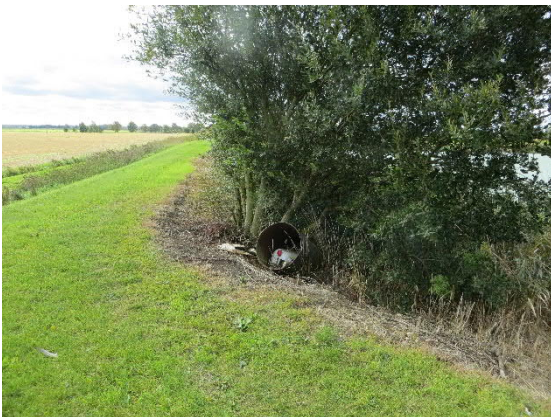
Figure 38: Example of “Satisfactory” Condition (Anglian Region)
