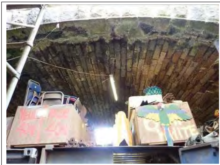
Photograph no 2: general view of the soffit
