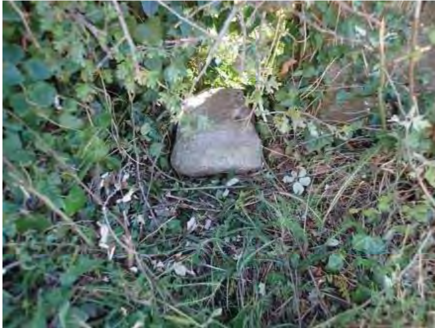
Photograph 21: the failed stone was placed adjacent to the U/S return of the parapet
