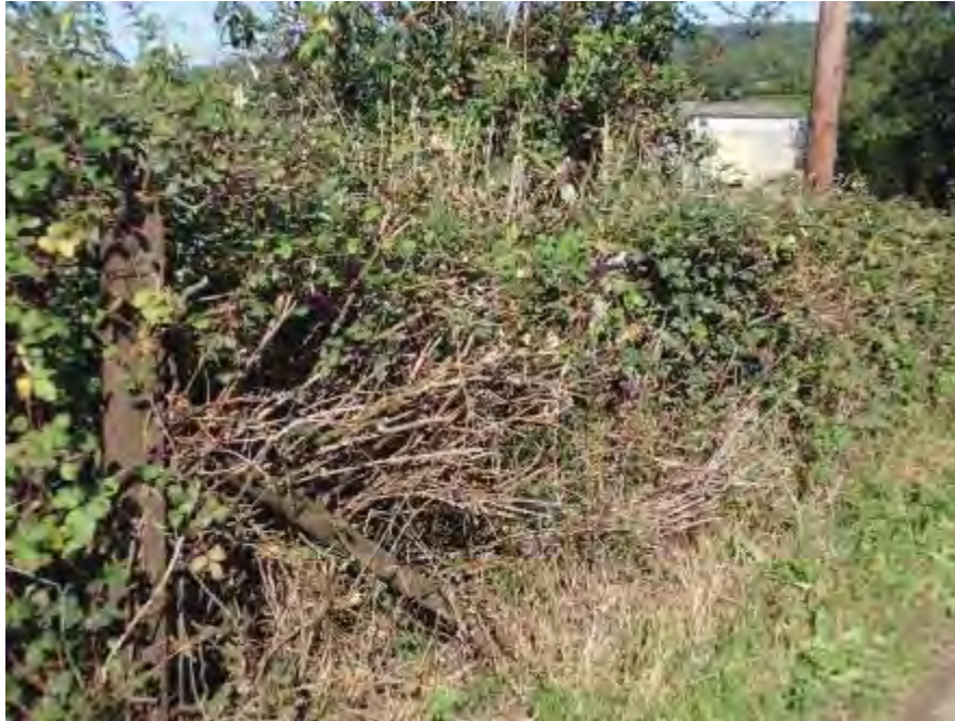
Photograph 43: long-standing failure of straining wires noted to the U/S, C/e approach fence
