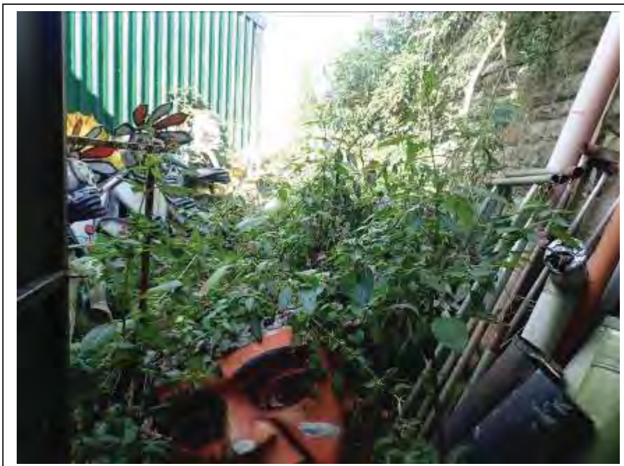
Photograph no 24: Himalayan Balsam located in front of the U/S, C/e wingwall
