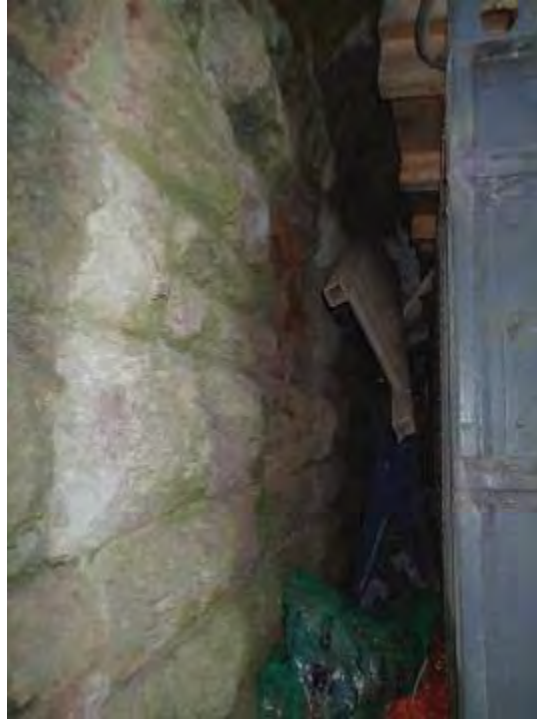
Photograph 3: general view of the U/S abutment
