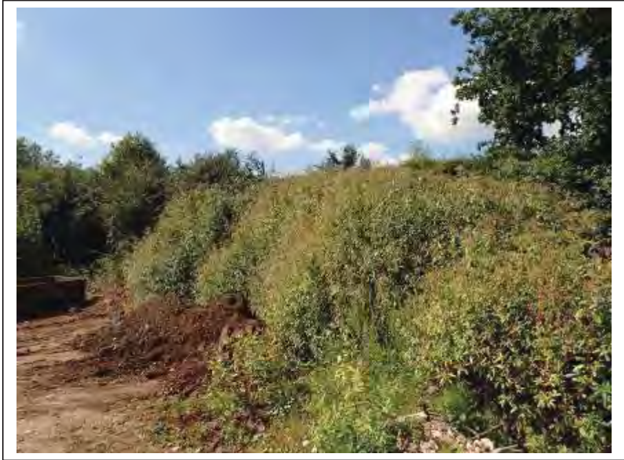
Photograph no 5: dense vegetation restricts access to the L/e elevation.
