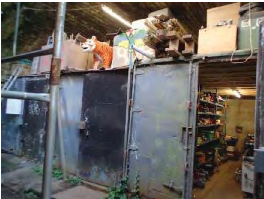
Photograph 46: metal storage containers below the structure restrict access
