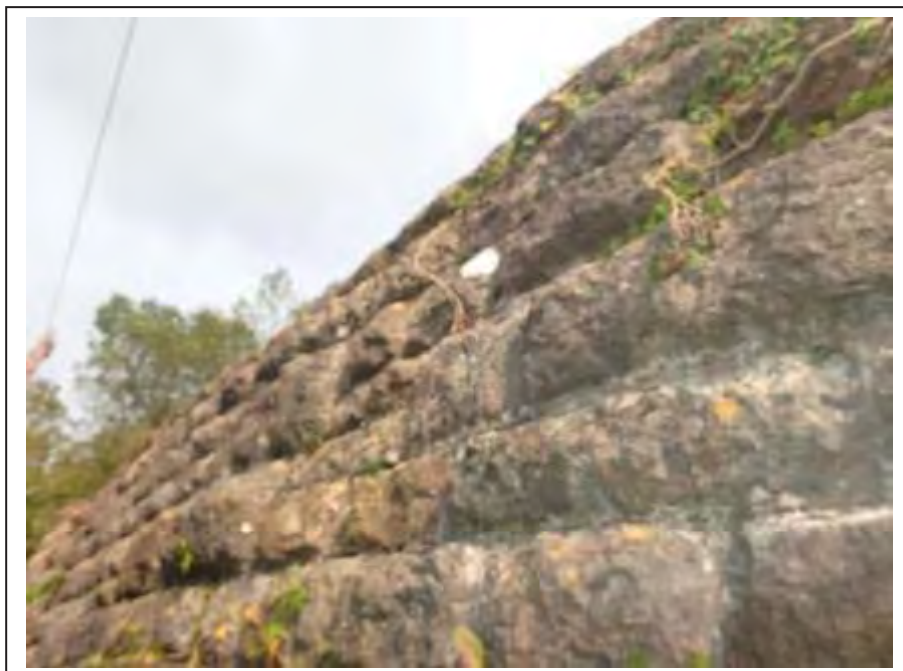
Photograph no 12: external face of the C/e parapet
