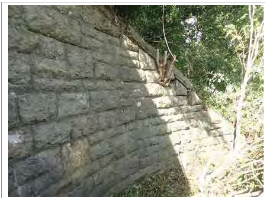
Photograph no 6: U/S, L/e wingwall
