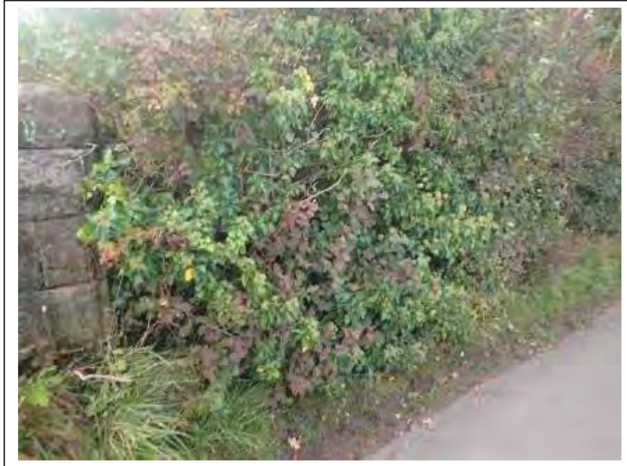
Photograph no 83: no fence line visible on the D/S, L/e
