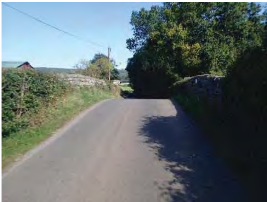
Photograph 10: general view over the structure from the D/S
