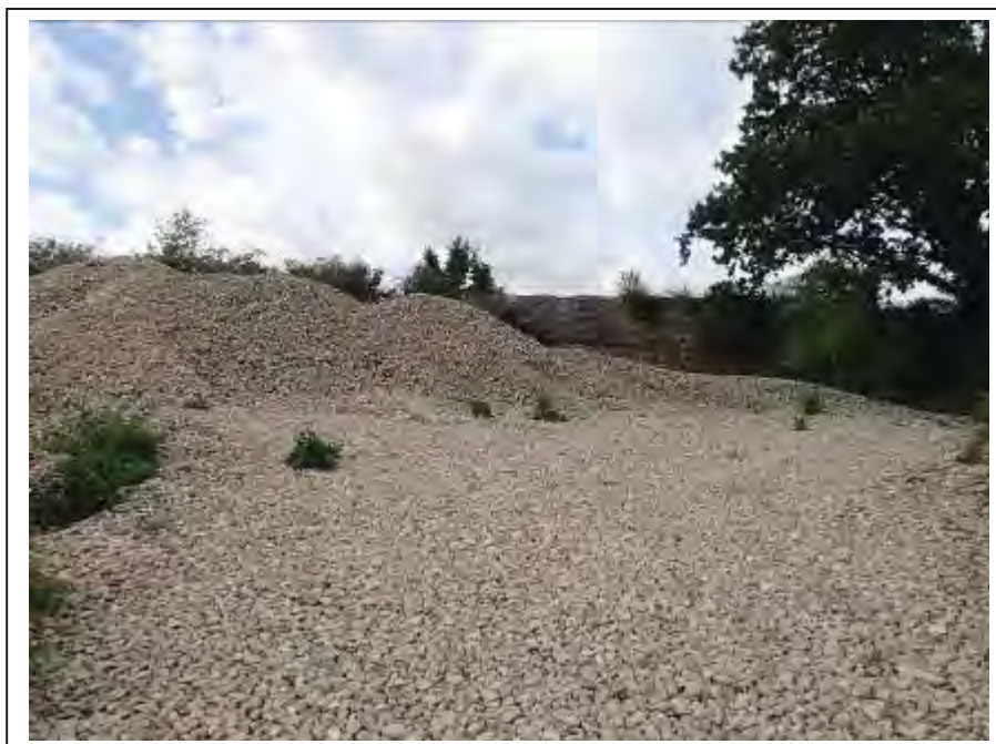
Photograph no 22: stone installed in front of the structure on the L/e
