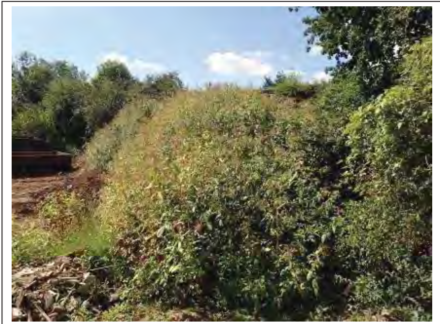
Photograph no 6: dense vegetation restricts access to the L/e elevation.
