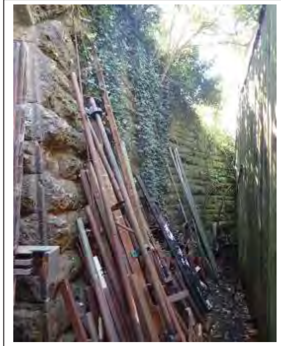
Photograph no 25: general view of the D/S, C/e wingwall
