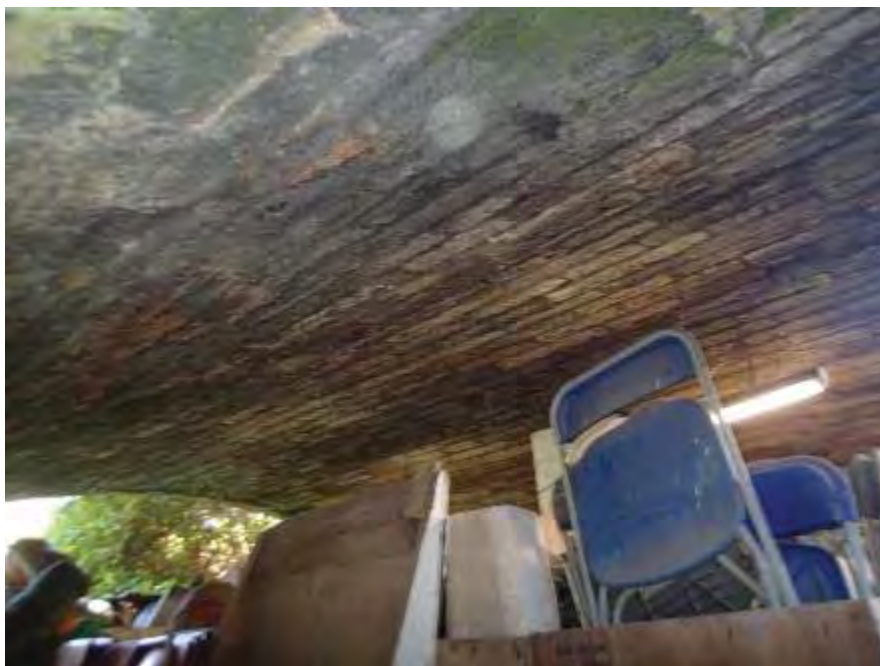
Photograph 2: general view of the soffit
