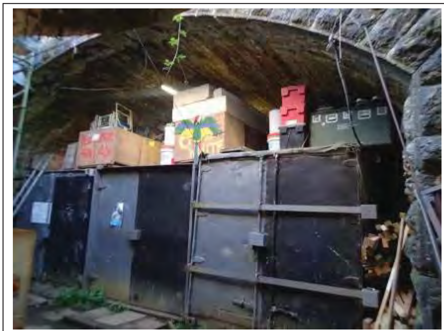
Photograph no 16: no access to the abutments
