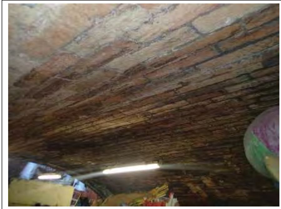
Photograph no 3: general view of the soffit
