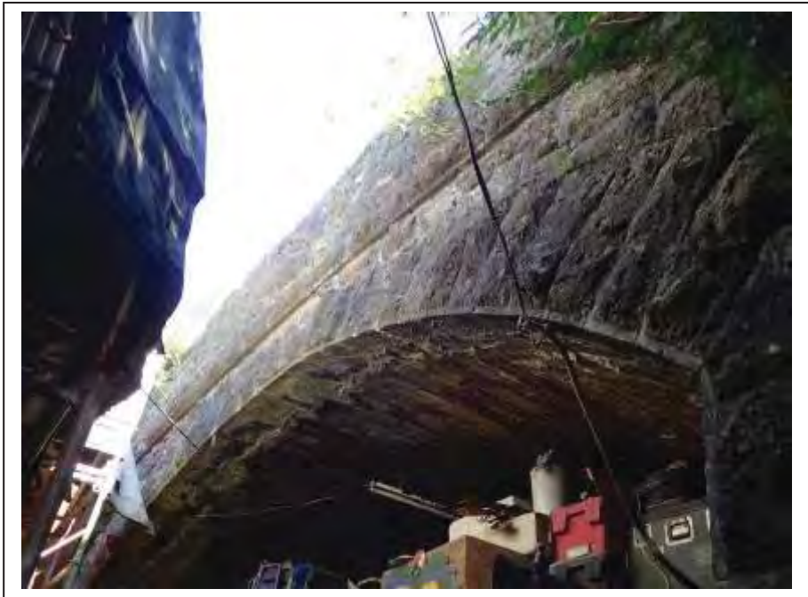
Photograph no 8: general condition of the C/e voussoirs
