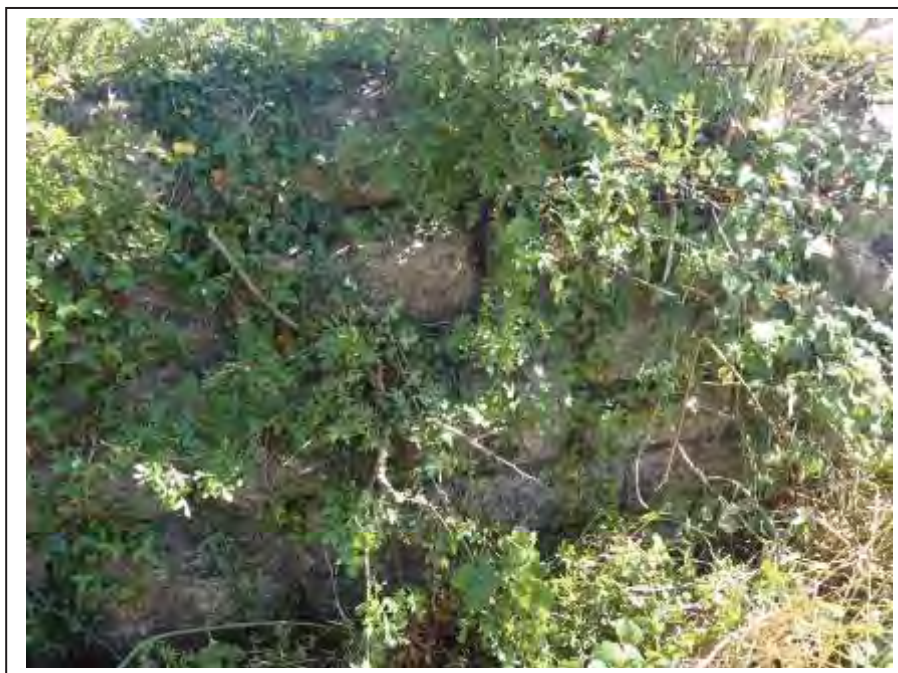
Photograph no 16: displaced copings along the L/e parapet located approx 2.7m from the U/S quoin
