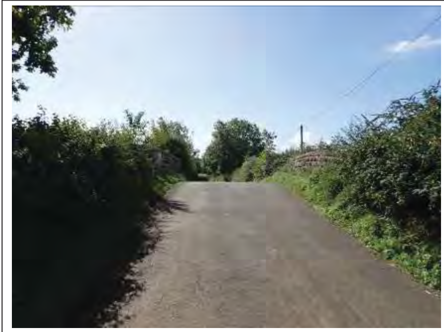
Photograph no 9: general view over the structure from the U/S
