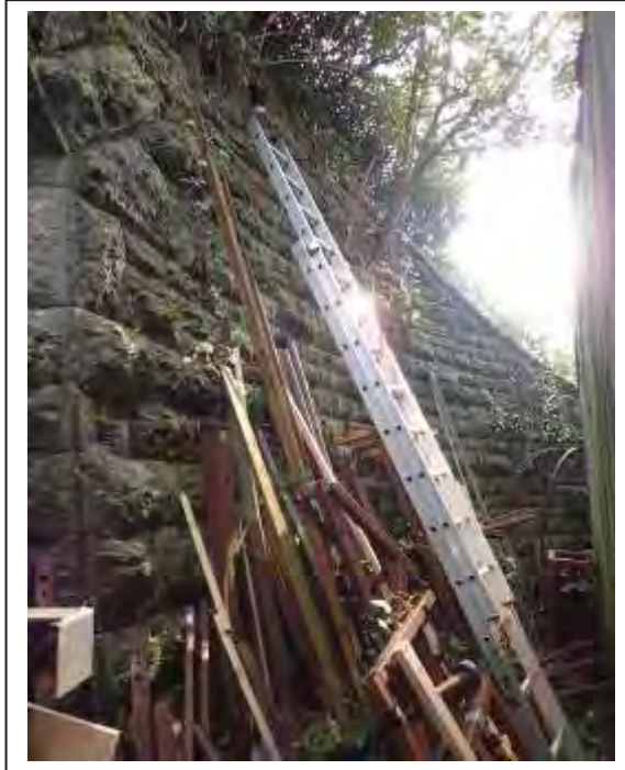
Photograph no 9: D/S, C/e wingwall
