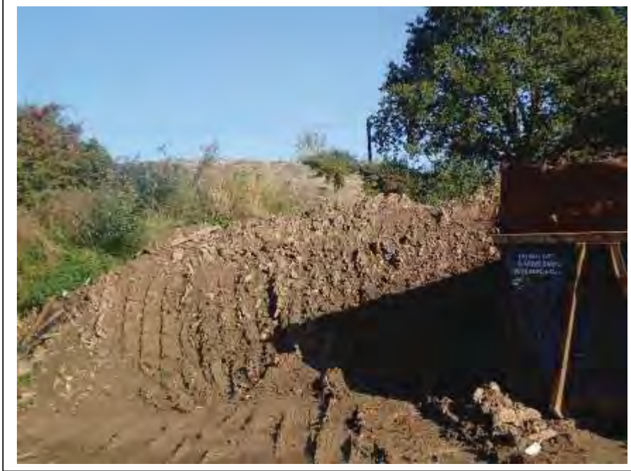
Photograph no 21: structure located behind stored materials on the L/e.
