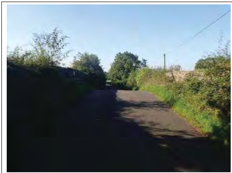
Photograph no 4: general view over the structure
