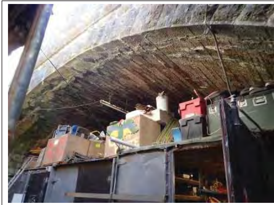
Photograph no 3: general view of the soffit
