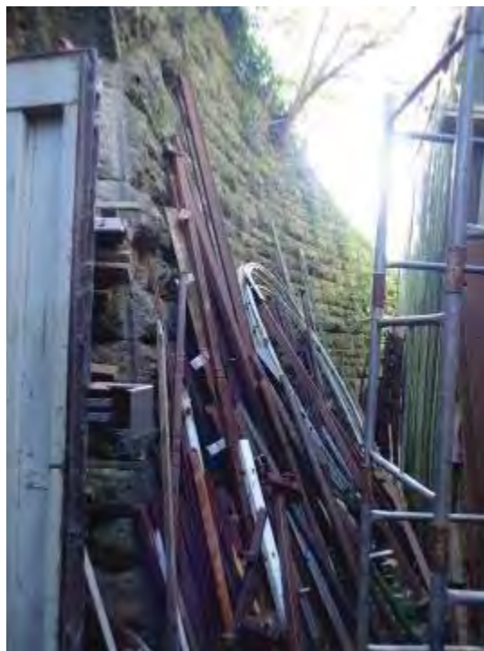
Photograph 8: general view of the D/S, C/e wingwall Stored materials restrict access to the wingwall
