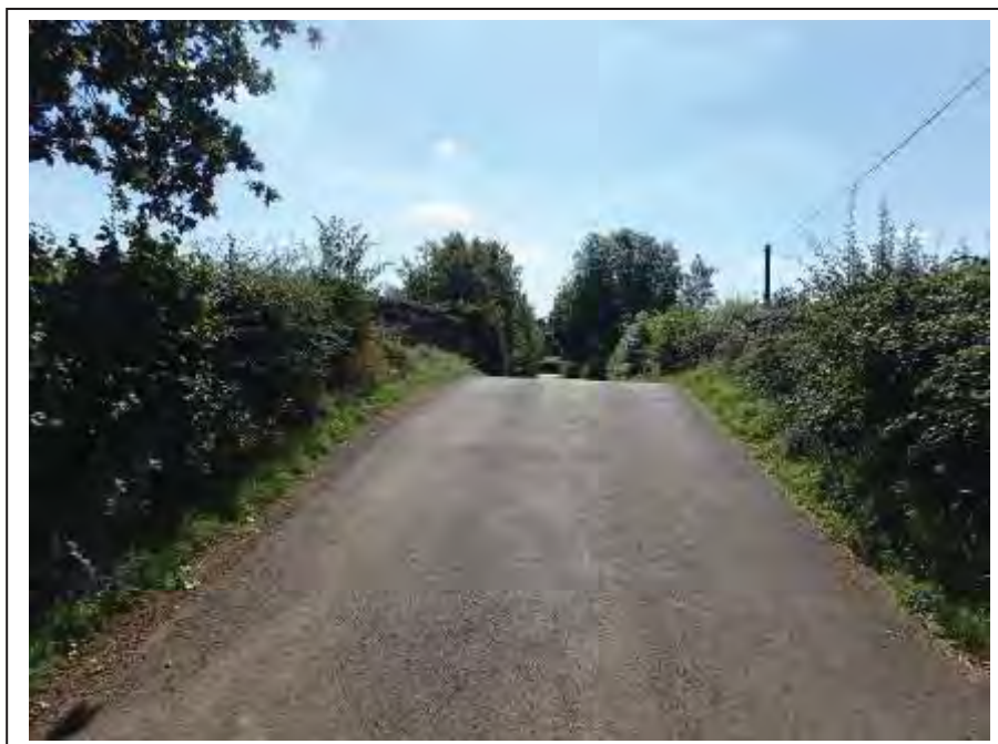
Photograph no 4: general view over the structure from the U/S
