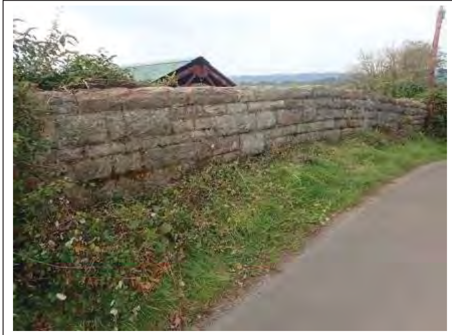
Photograph no 13: internal face of the C/e parapet
