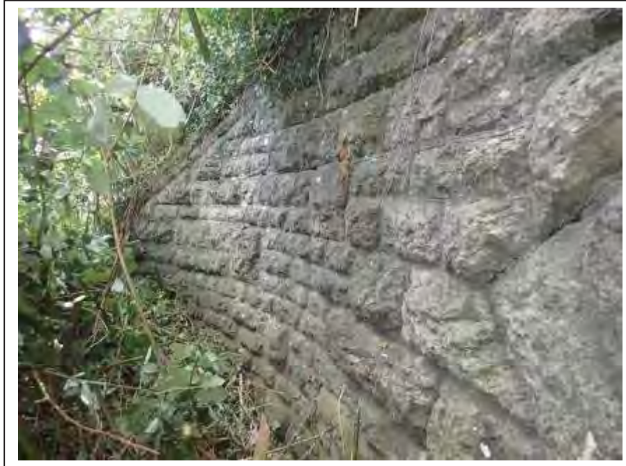
Photograph no 7: D/S, L/e wingwall
