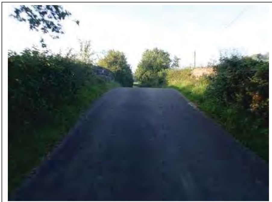
Photograph no 2: general view over the structure
