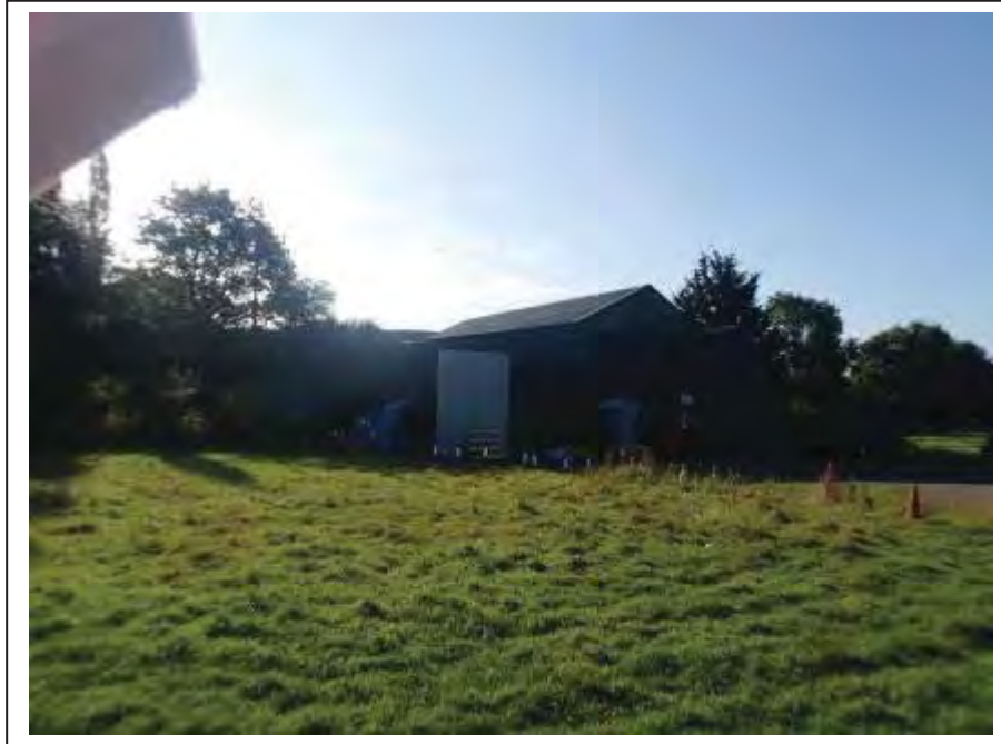
Photograph no 1: Country elevation The structure is covered from view by installed buildings.
