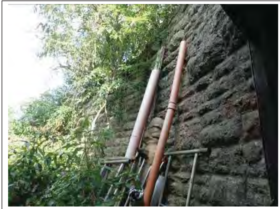
Photograph no 7: general view of the U/S, C/e wingwall
