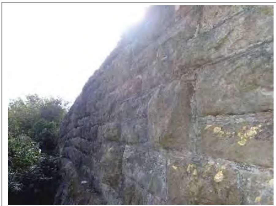
Photograph no 10: external face of the L/e parapet
