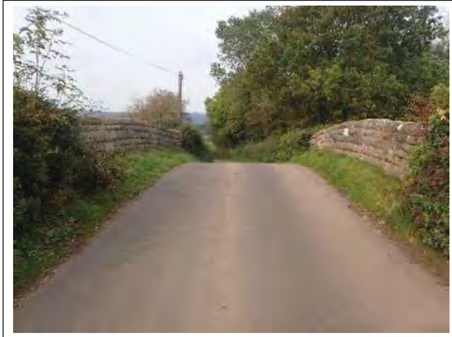
Photograph no 15: general view over the structure from the D/S
