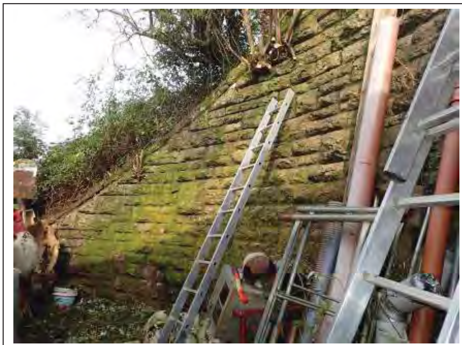
Photograph no 8: U/S, C/e wingwall
