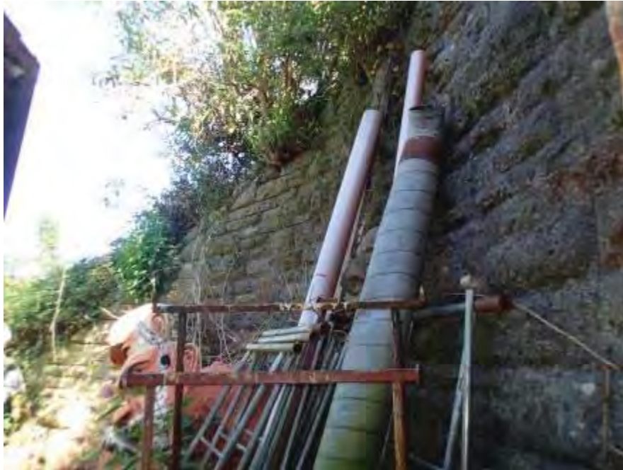
Photograph 7: general view of the U/S, C/e wingwall
