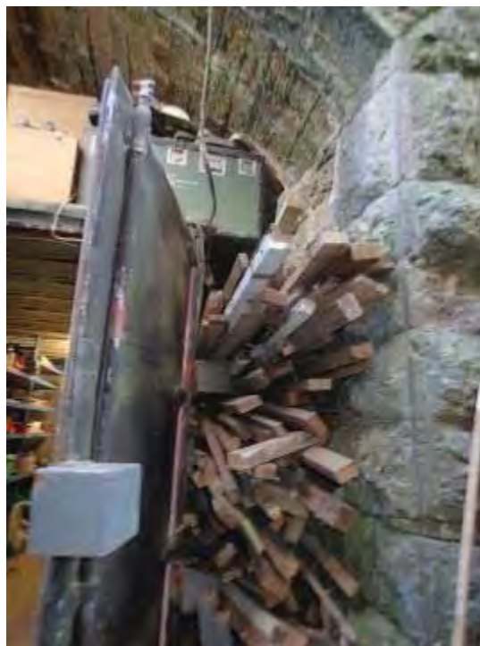
Photograph 4: general view of the D/S abutment
