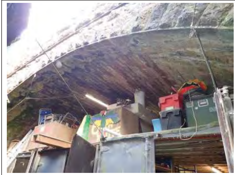
Photograph no 5: general view of the soffit
