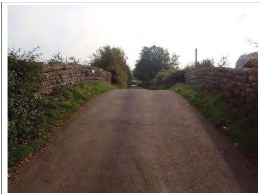
Photograph no 14: general view over the structure from the U/S
