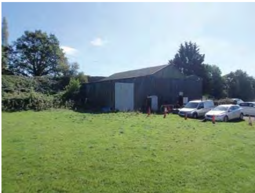
Photograph 48: work shed located in front of the structure on the C/e
