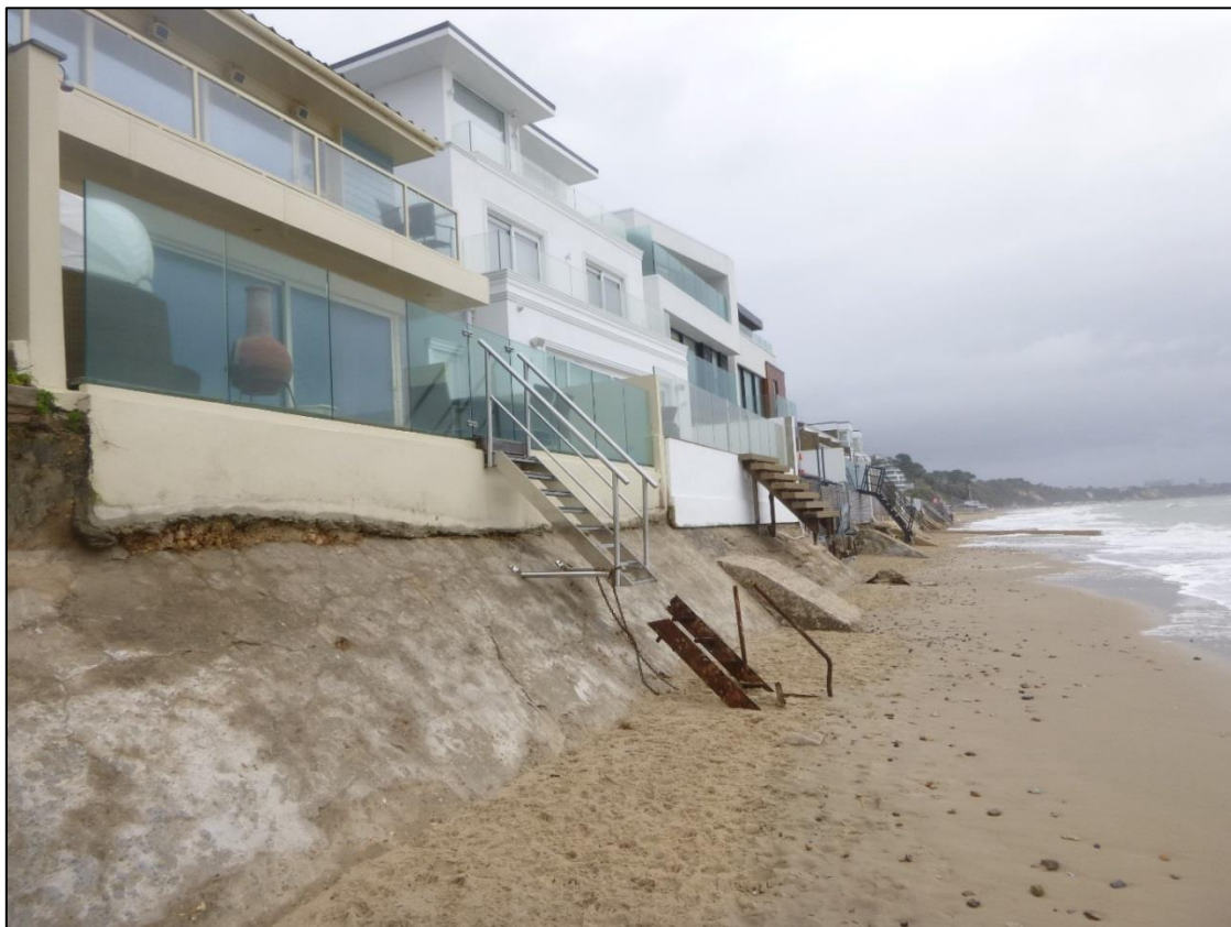
Figure B.1 Beach erosion at Sandbanks following the winter 2013 to 2014 storms left the beach denuded of sand
