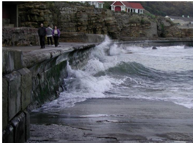
Figure 3.10 Example of wave loading on a structure (seawall)
