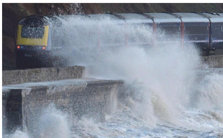
Figure 3.7 Wave overtopping onto a moving train, UK
