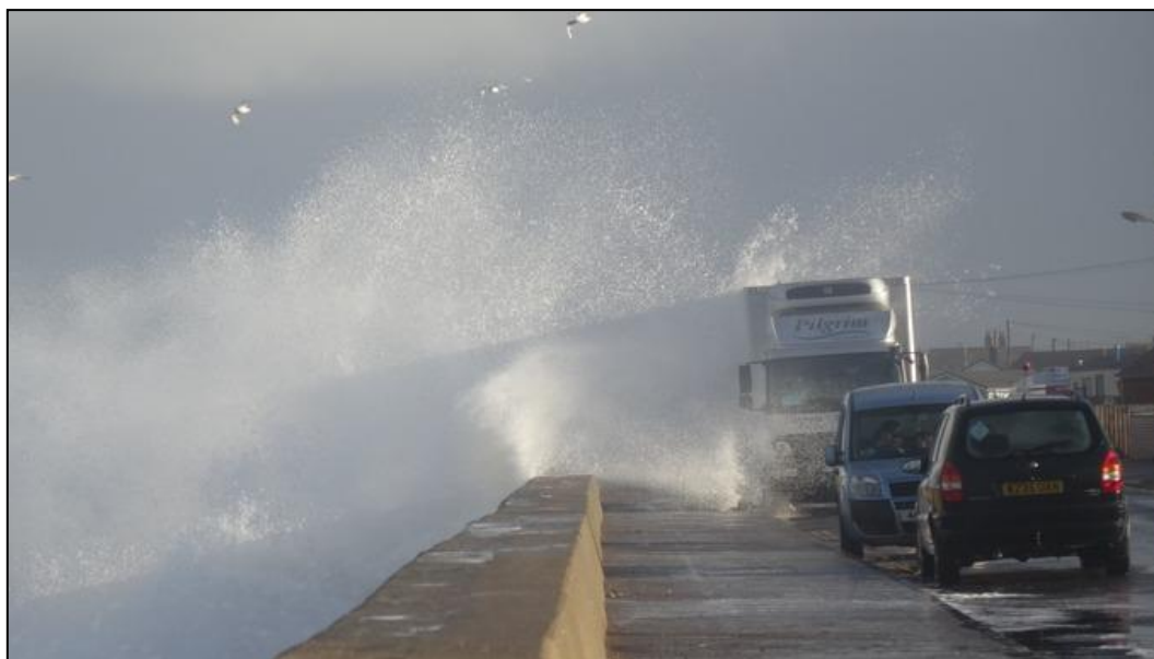
Figure 4.42 Wave overtopping at Walcott in 2013
