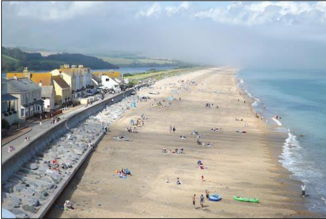
Figure 4.33 Photograph taken looking north across the beach at Torcross
