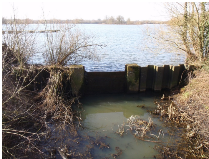
Figure 2.3 Stop logs used for drawdown capability at a low dam
