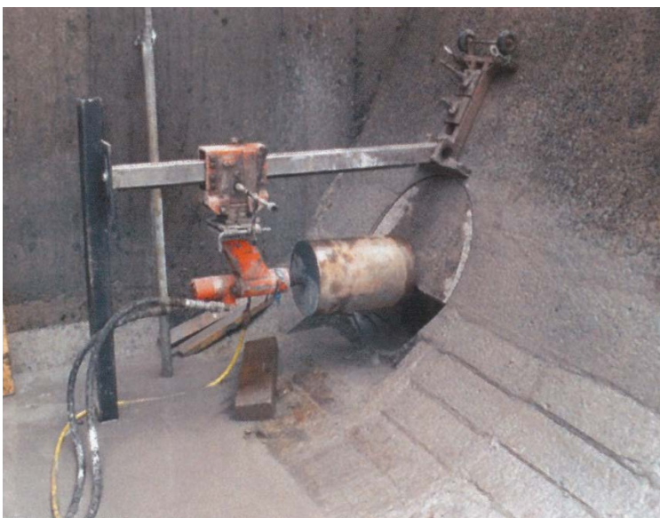
Figure 2.2 Outlet being retrofitted through spillway weir wall (Northern Ireland Water, 2014(b))
