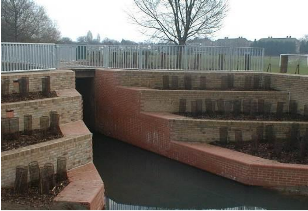
Figure 3.9 Flume control on a walled flood control dam
