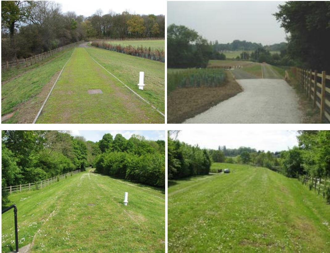
Figure 3.4 Example of tree screening: Radlett flood storage reservoir in 2005 and 2014
