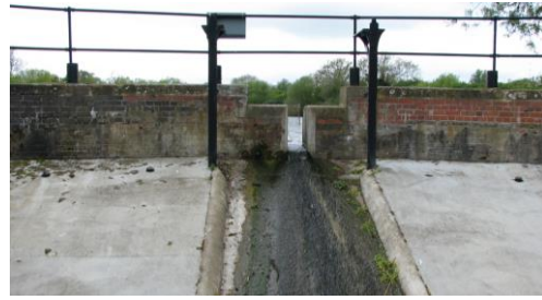
(b) Overflow showing 1,500mm wide notch and 300mm wide slot
