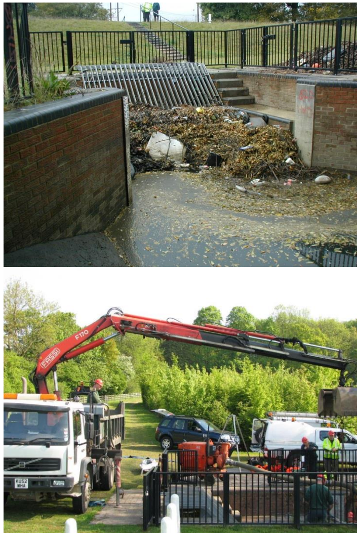
Figure 3.13 Screen design allows for manual raking or cleaning by grab lorry
