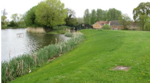
(c) Upstream face of dam, showing good reed margin and proximity of residential development
