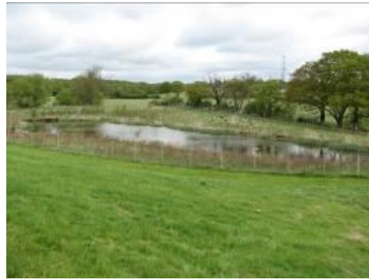
(b) Cobbins Brook borrow area reinstated as a wetland pond. The photograph was taken in May 2013 following establishment of the site.
