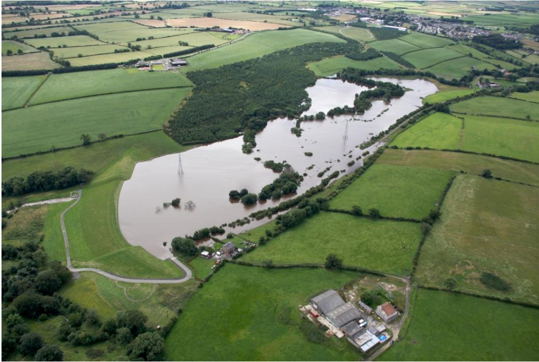
Figure 2.6 Spring Gardens flood storage reservoir: an example of an impounded online flood storage reservoir
