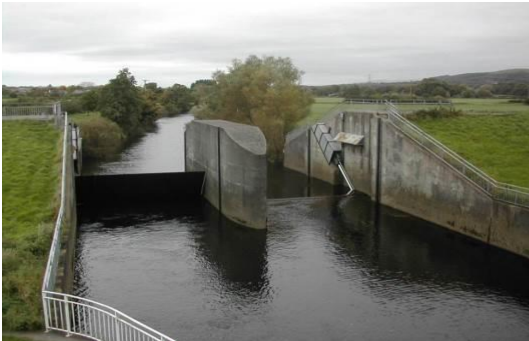
Figure 4.4 Online overshoot radial gate being raised from the watercourse bed
