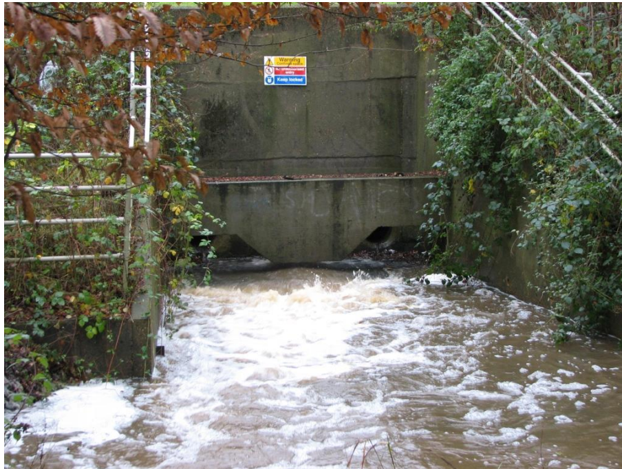
Figure C.1 Example of USBR impact-type basin
