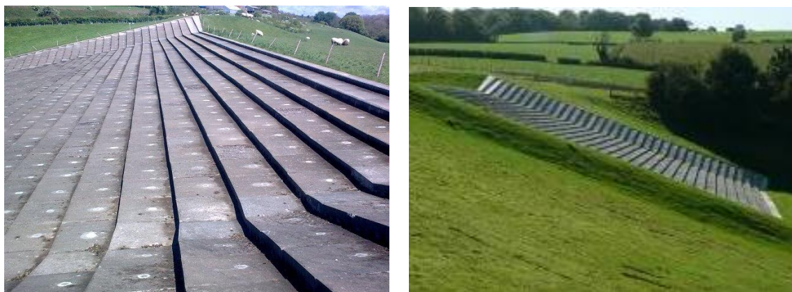
Figure B.7 Examples of wedge-block spillways
