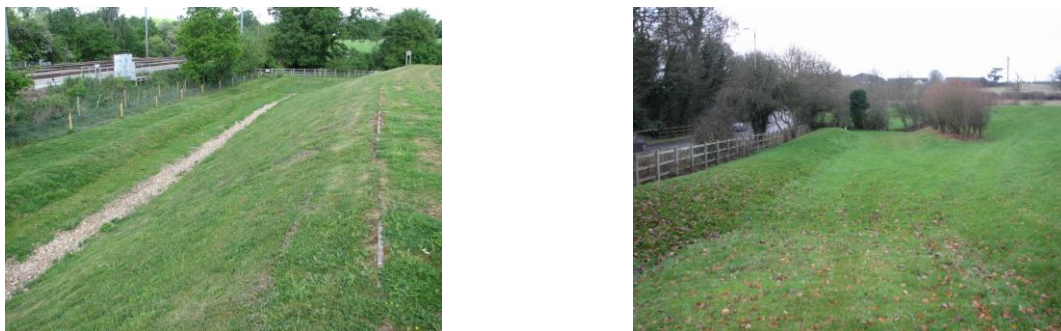
Figure 2.9 Examples of training bunds to protect rail and road infrastructure Photographs courtesy of ATPEC Ltd
