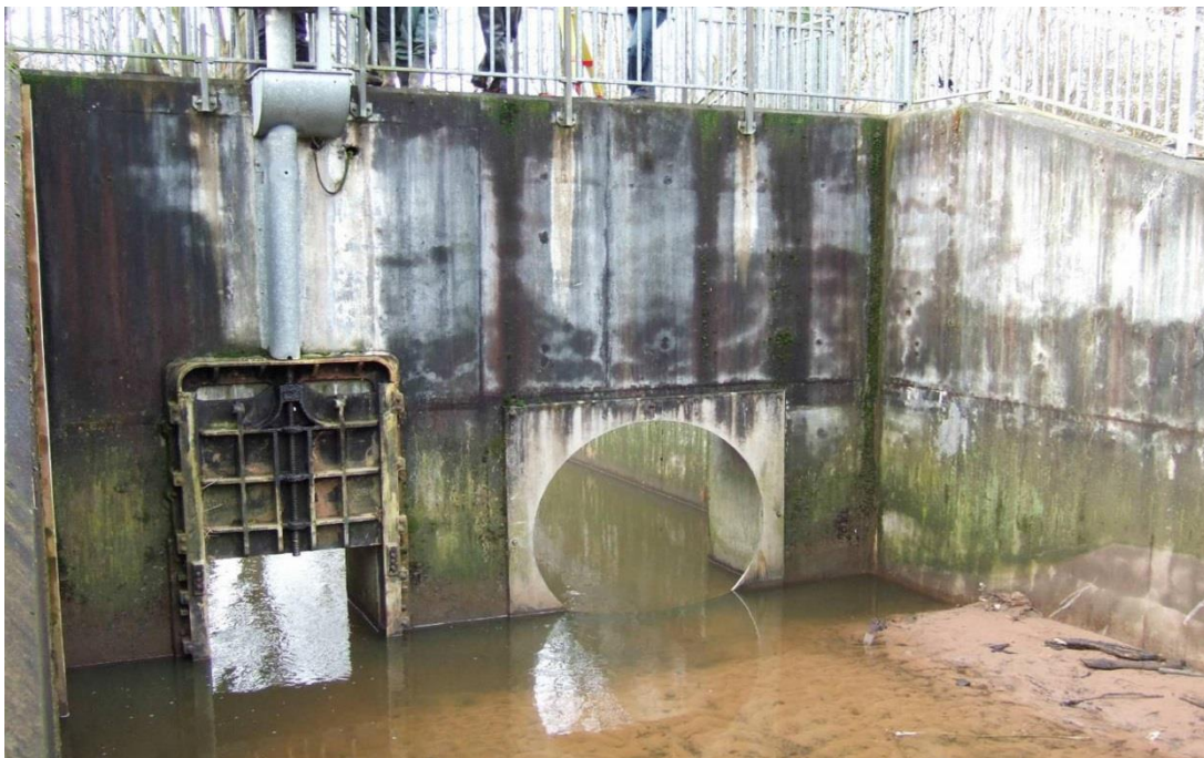
Figure 4.5 Orifice plate and supplementary control penstock
