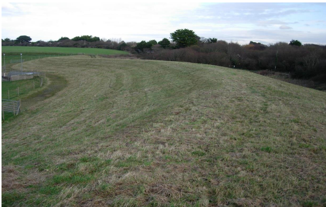
Figure 3.18 Short grass provides for effective surveillance of embankment condition
